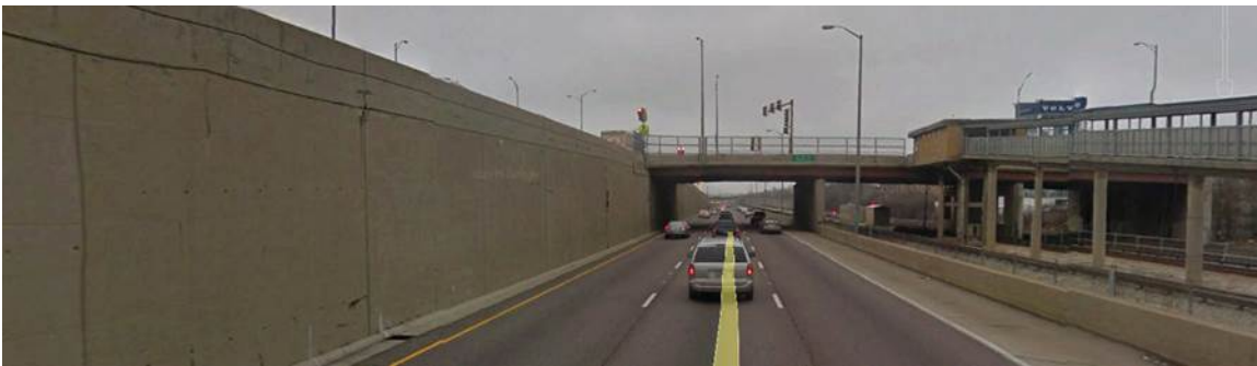
View of eastbound I-290's center on/off ramp walls (at left) and CTA facilities (at right) at Harlem Avenue.
