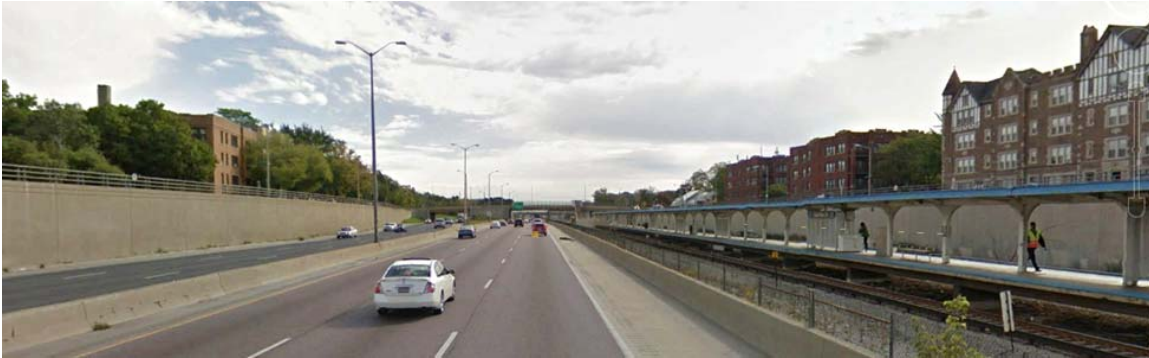
View of I-290's retaining walls (at left), CTA facilities and mid-rise adjacent housing structures (at right) east of South Oak Park Avenue.
