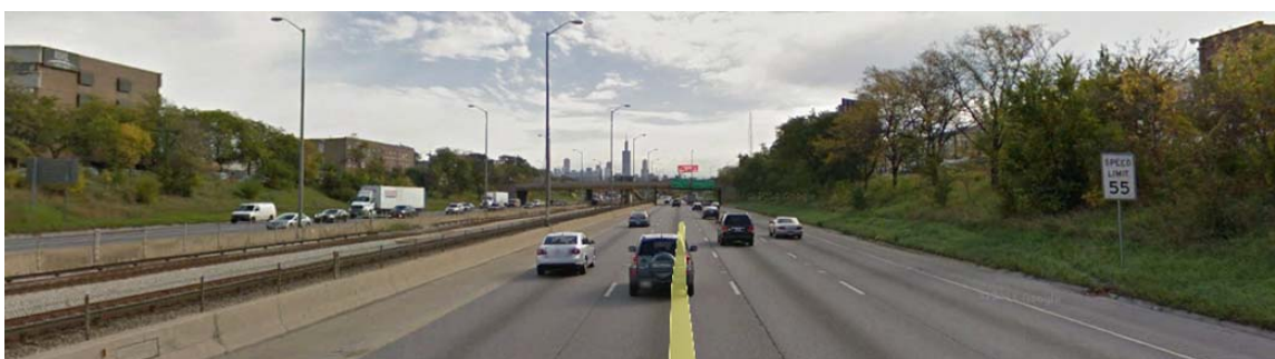
View of I-290 Project Corridor east of South Central Park Avenue.
