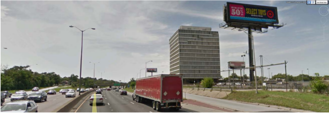
View of I-290 Project Corridor proximate to the northeast quadrant of the I-290/1 st Avenue interchange.
