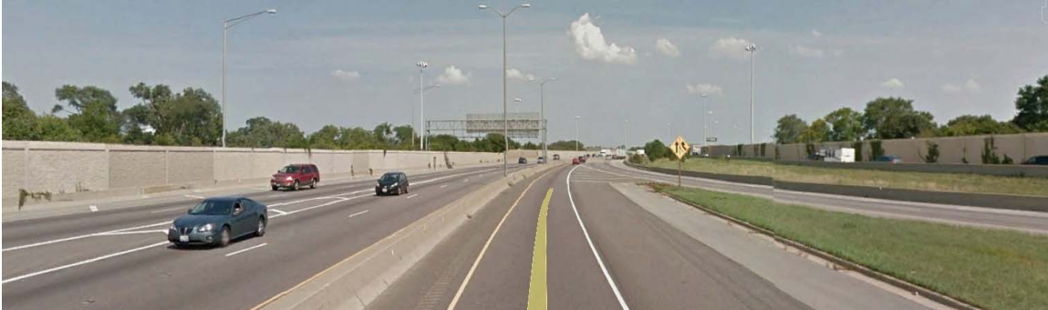
View of existing noise barriers between I-290 and adjacent residential neighborhoods in the western portion of the Study Area.
