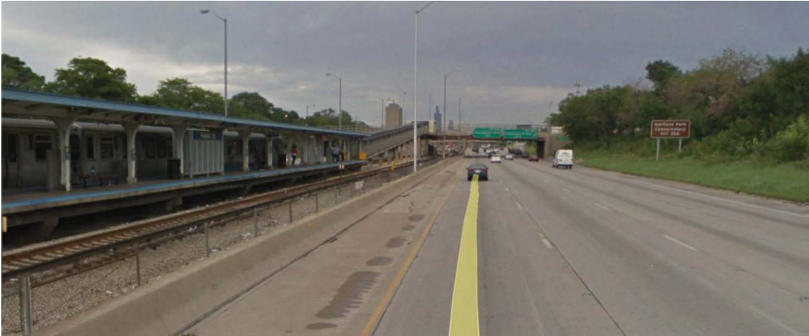
View of I-290 Project Corridor eastbound lanes (at right) and CTA facilities in median (at left) east of South Laramie Avenue.
