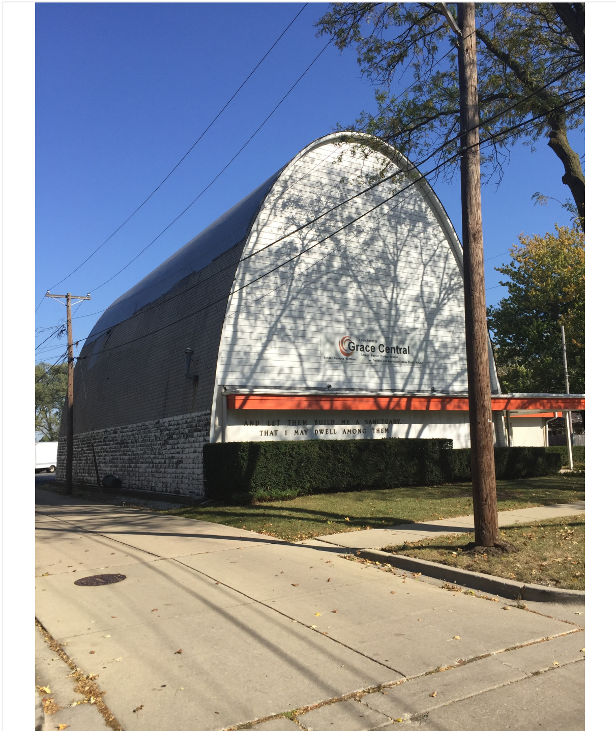
Facing northeast to the south facade and west elevation from Kitchner Street
