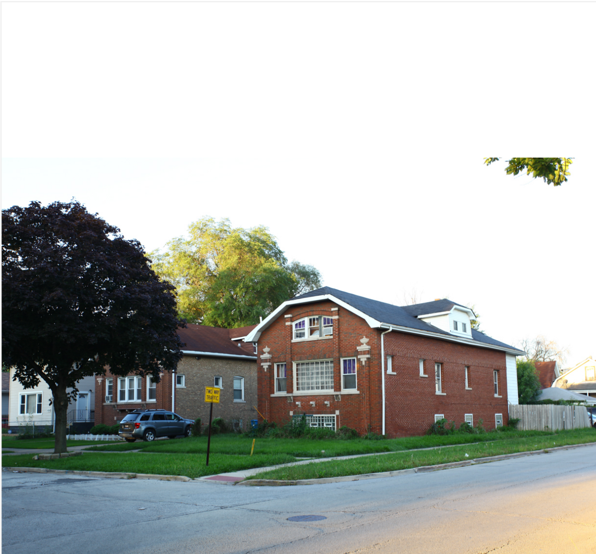
Photo 2 - 1818 South 7th Avenue
