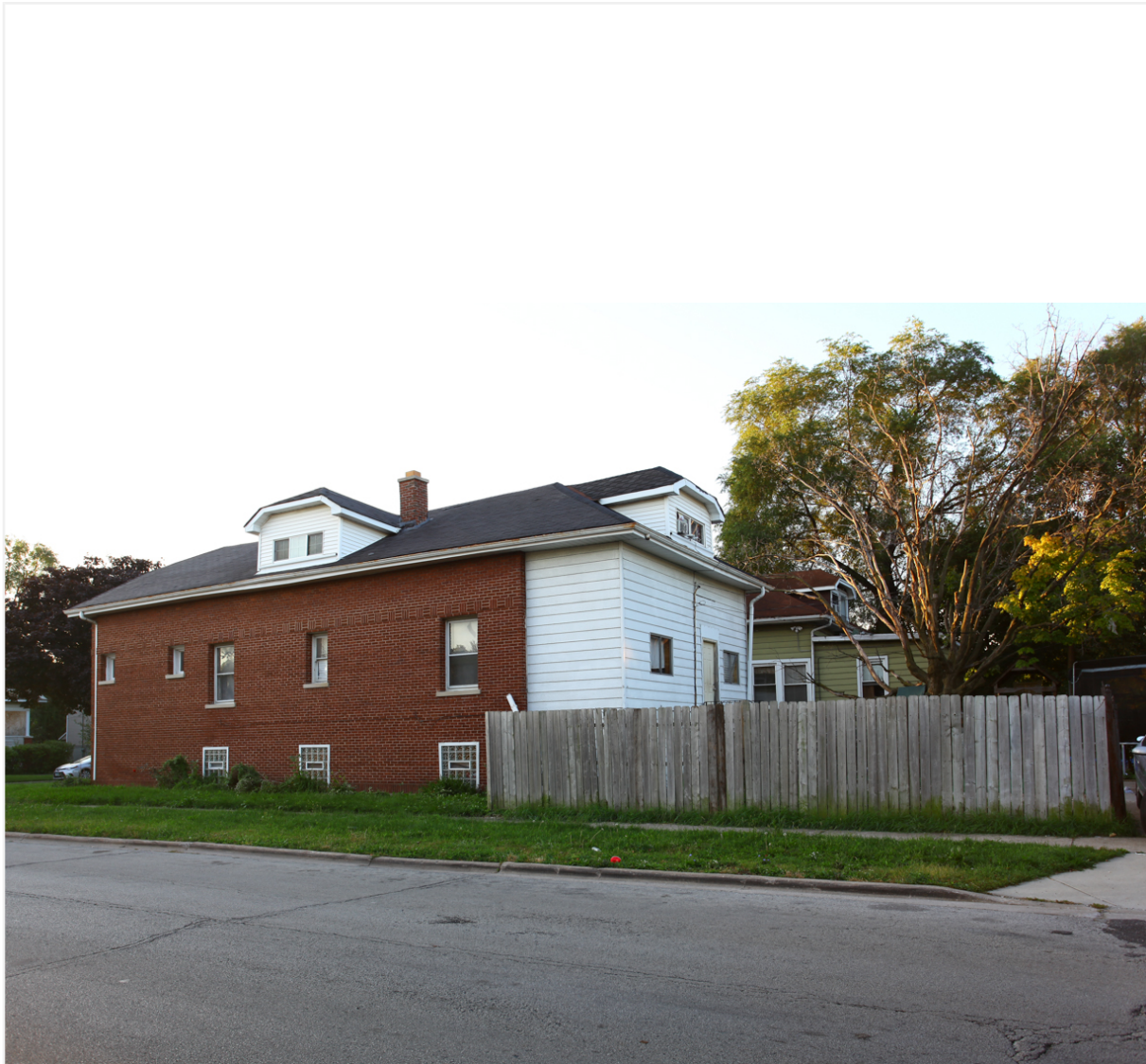
Photo 4 - 1818 South 7th Avenue
