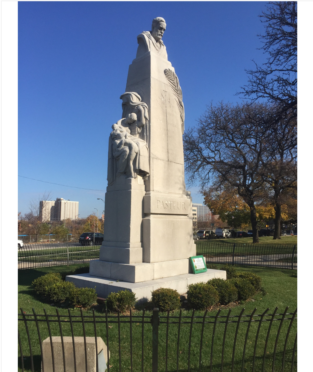
Facing northwest to south and west sides of monument from within green space
