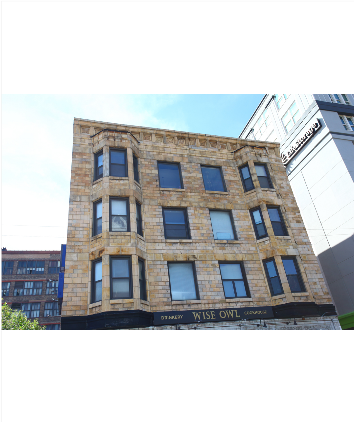
Close-up view of west-facing facade's upper stories
