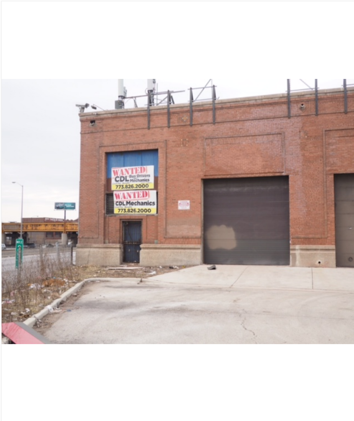
Facing west to east-facing facade of the ca. 1950 addition
