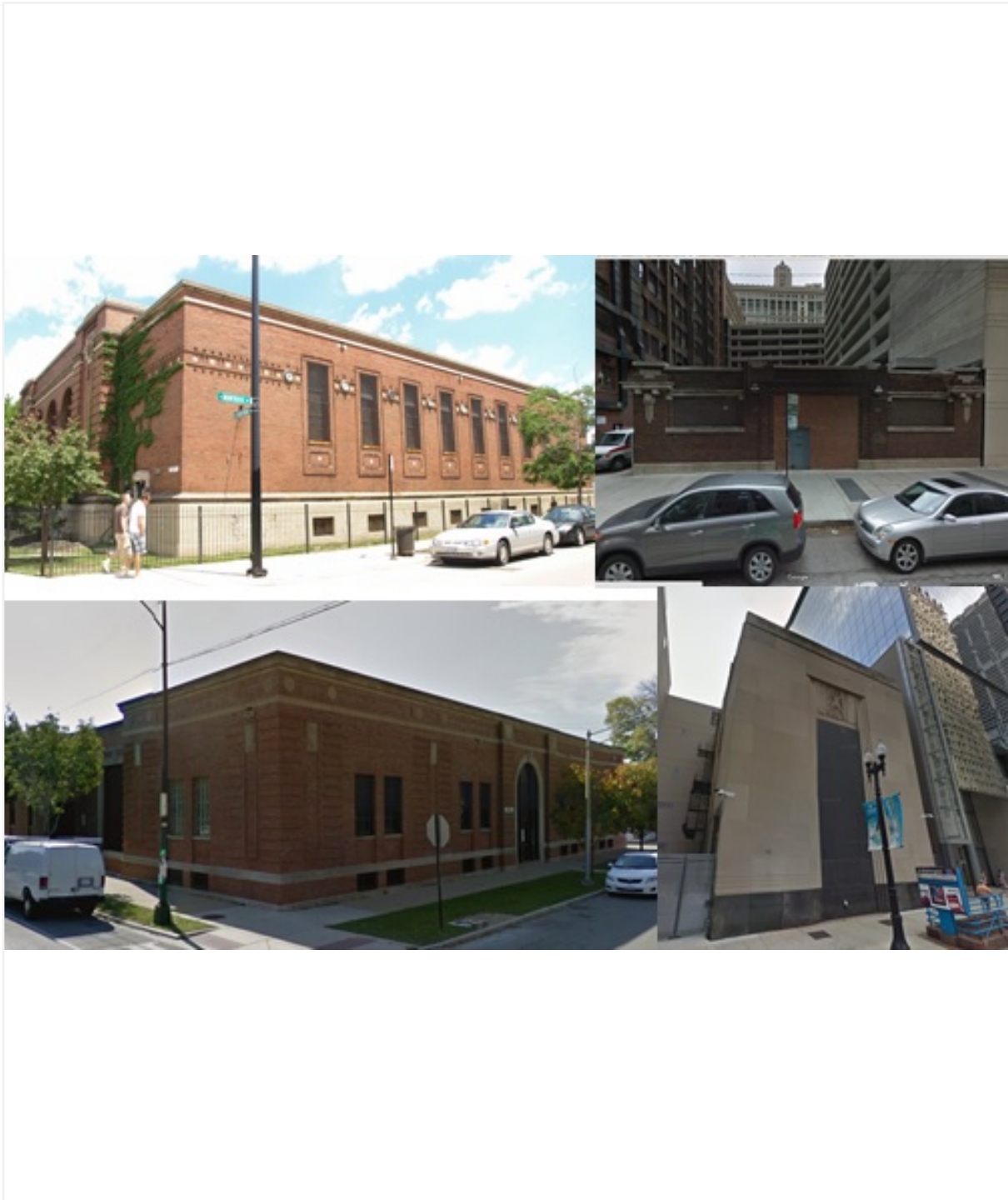
Top Left Photo: 4401 North Clifton Avenue (Cook County Assessor's Office); Top Right Photo: 321 South Franklin Avenue (Google Maps November 2015); Bottom Left Photo: 6405 West School Street; Bottom Right Photo: 115 North Dearborn Street
