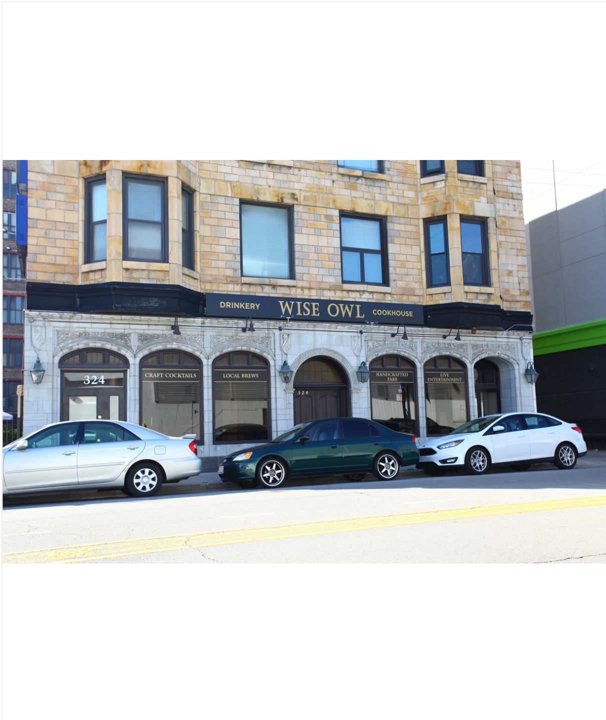
Close-up view of west-facing facade's first story
