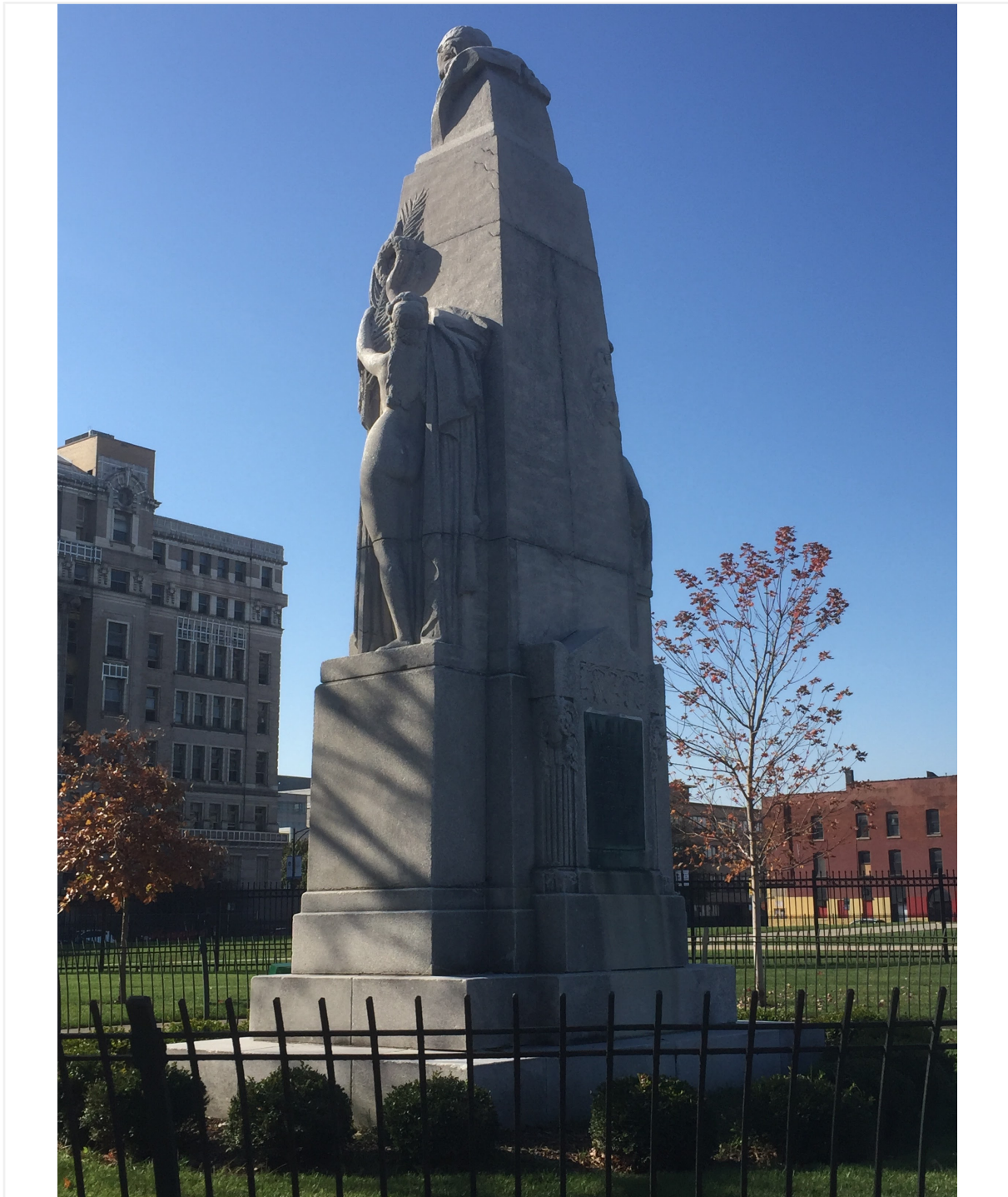
Facing southwest to north and east sides of monument from within green space, Cook County Hospital Administration Building visible at left
