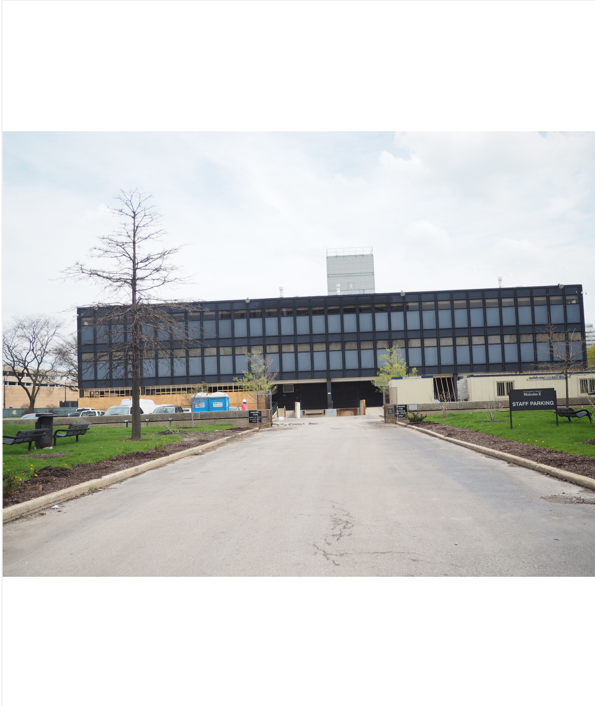
Facing east to west elevation from South Damen Avenue
