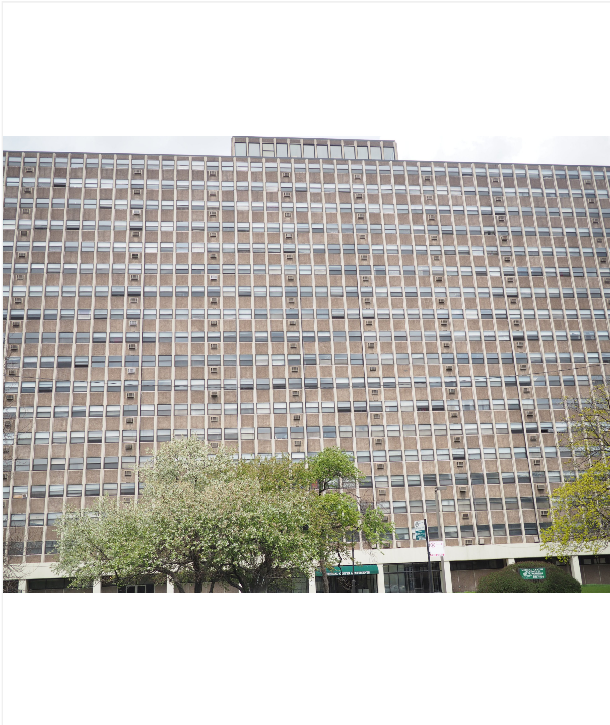
Facing north to south elevation from West Harrison Street
