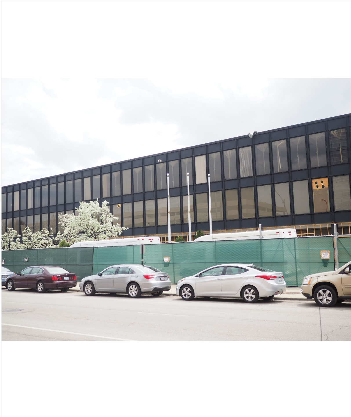
Facing south to north elevation from West Jackson Boulevard
