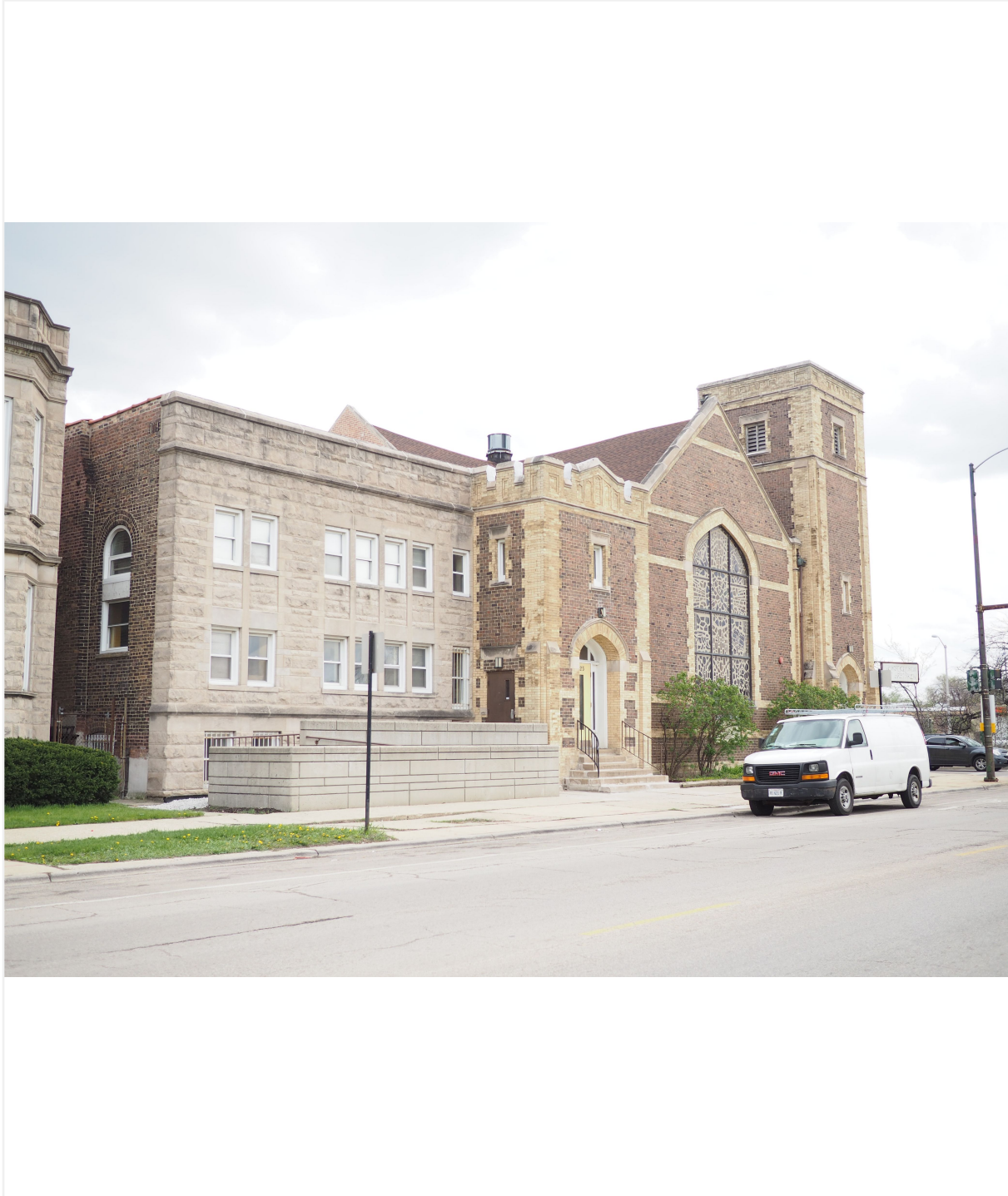
Facing southeast to west and north elevations from South Central Park Boulevard (two-flat visible at left)
