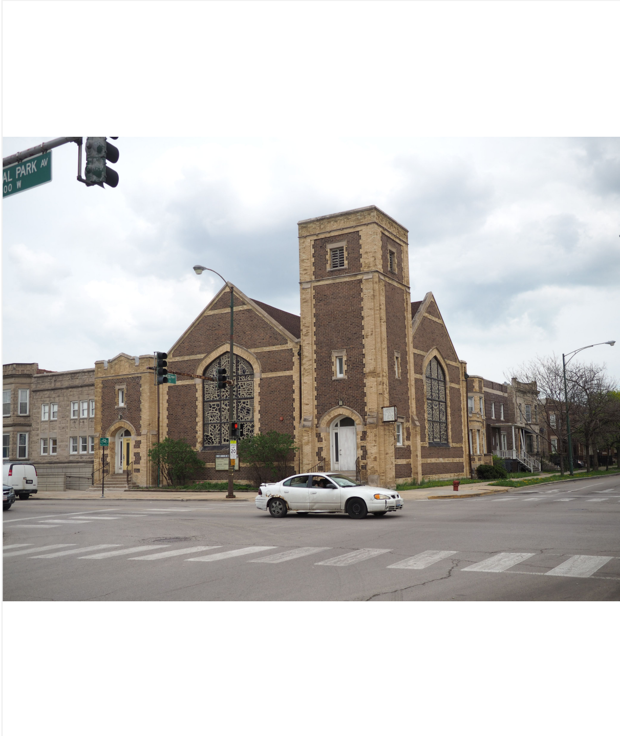
Facing northeast to south and west elevations from South Central Park Boulevard and West Congress Parkway
