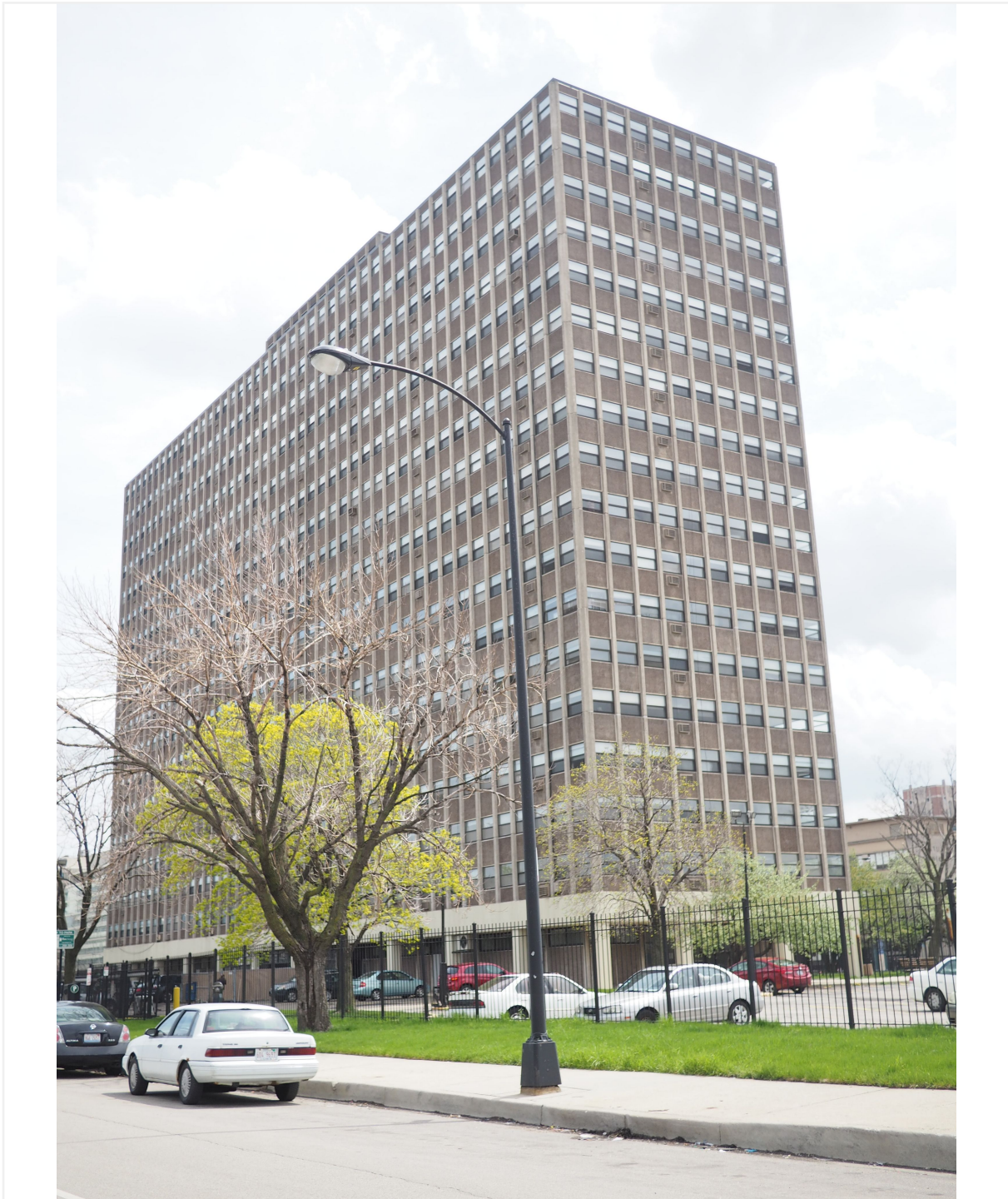
Facing southeast to west and north elevations from West Congress Parkway
