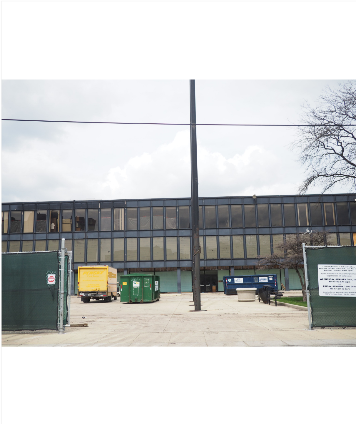
Facing north to south elevation from West Van Buren Street
