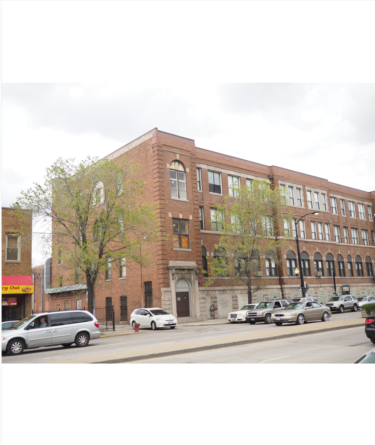
Facing northwest to south rear and east side elevations of main church and school building from South Western Avenue
