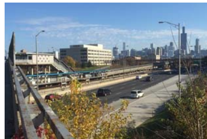
View northeast from Ogden Ave to I-290 near Louis Pasteur Memorial
