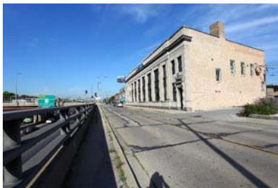
View west along Harrison St to Suburban Trust and Bank Building (R), S Oak Park Ave, & I-290 (L)
