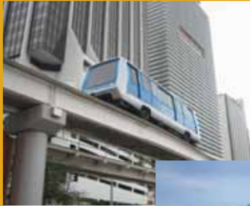
Automated Guideway Transit
