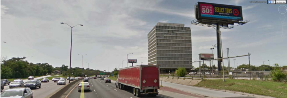
View of I-290 Project Corridor proximate to the northeast quadrant of the I-290/1 st Avenue interchange.
