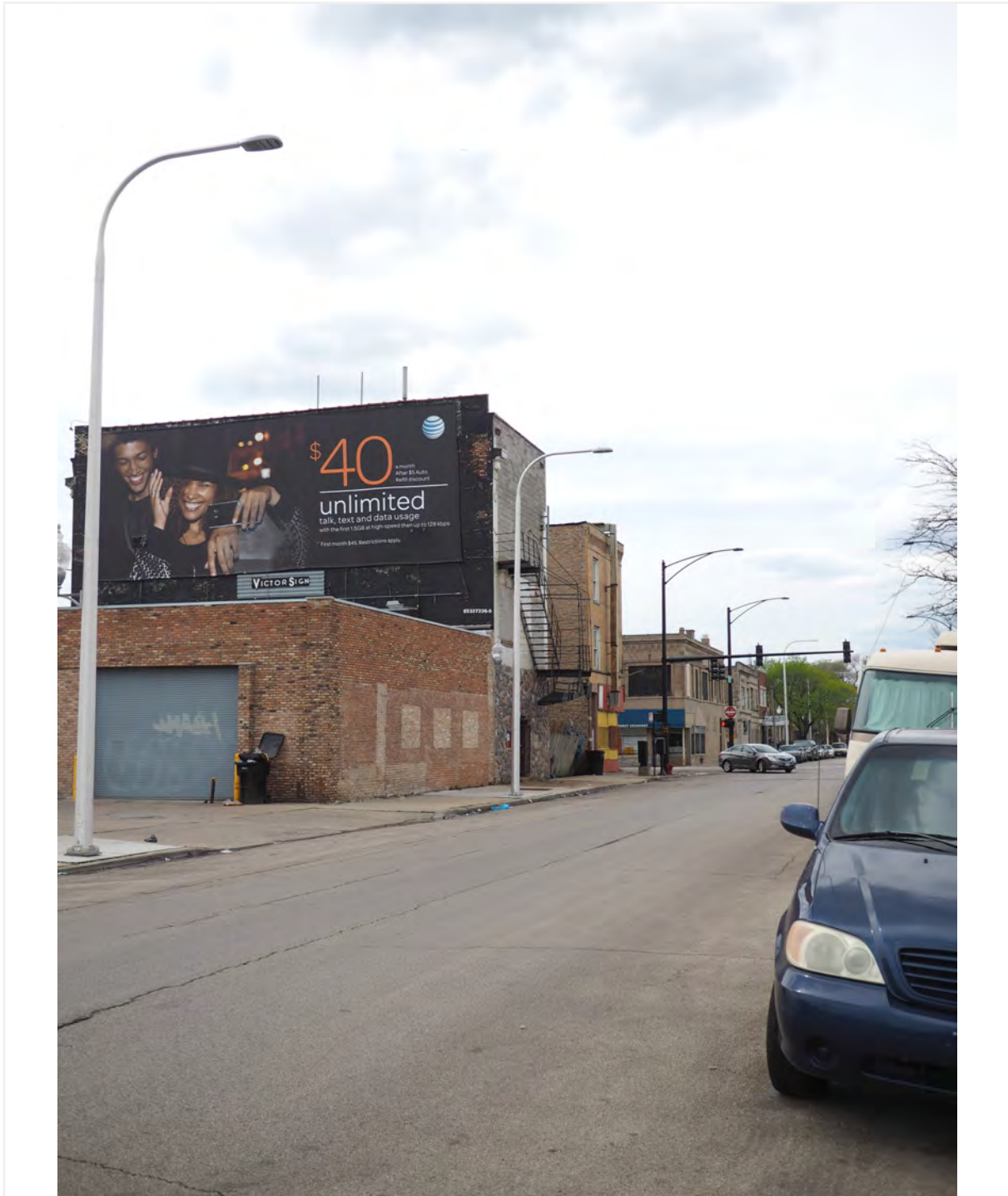
Facing southwest to commercial buildings at 3937, 3953, and 3959 West Harrison Street from West 5th Avenue (left to right)
