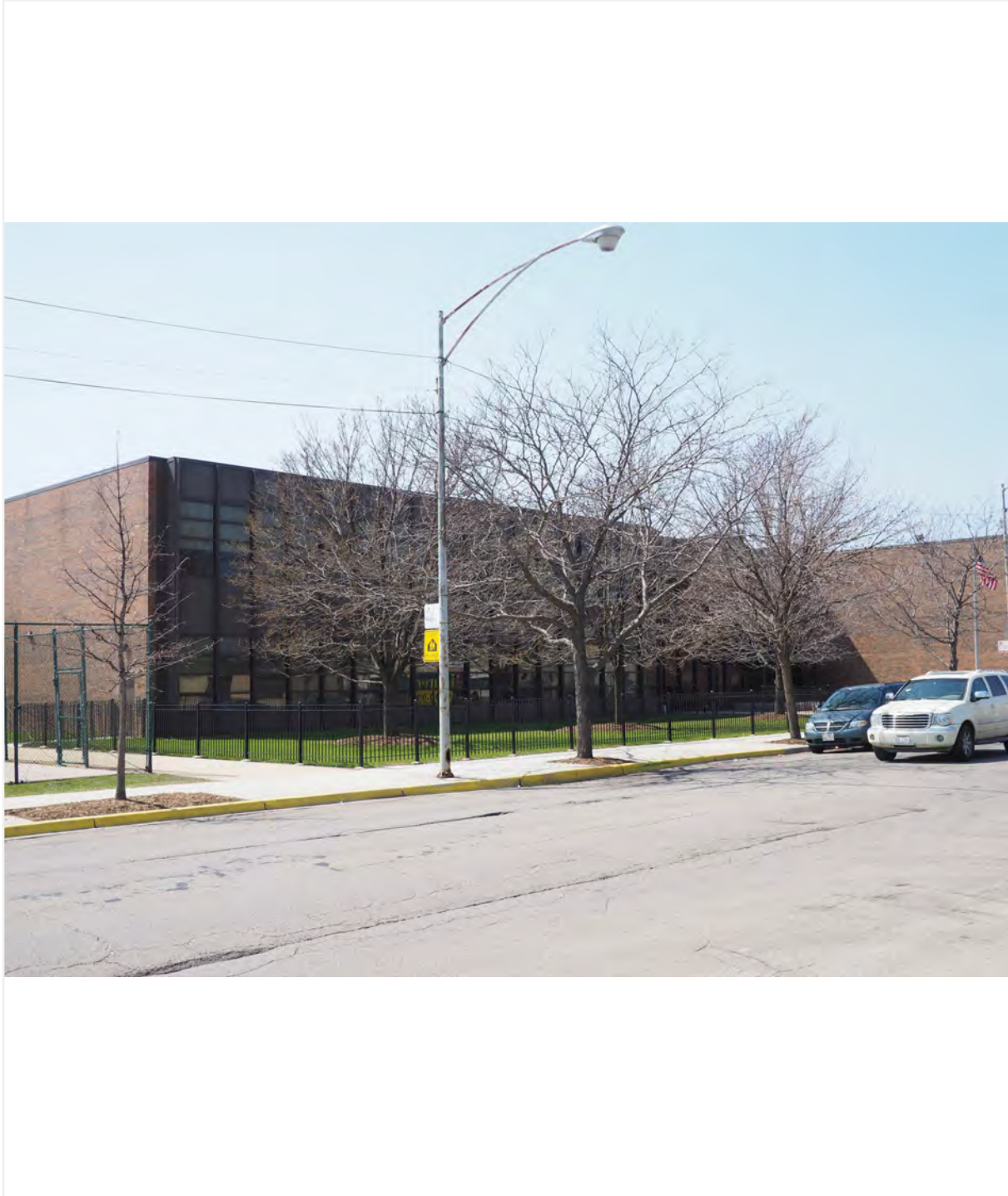
Facing southwest to north-facing facade and east side elevation from West Harrison Street
