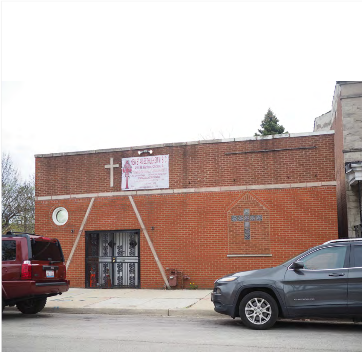
Photo 19 - West Harrison Street District
