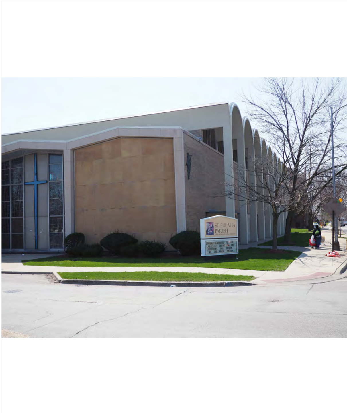
Facing south to north-facing facade and west side elevation from West Bataan Drive
