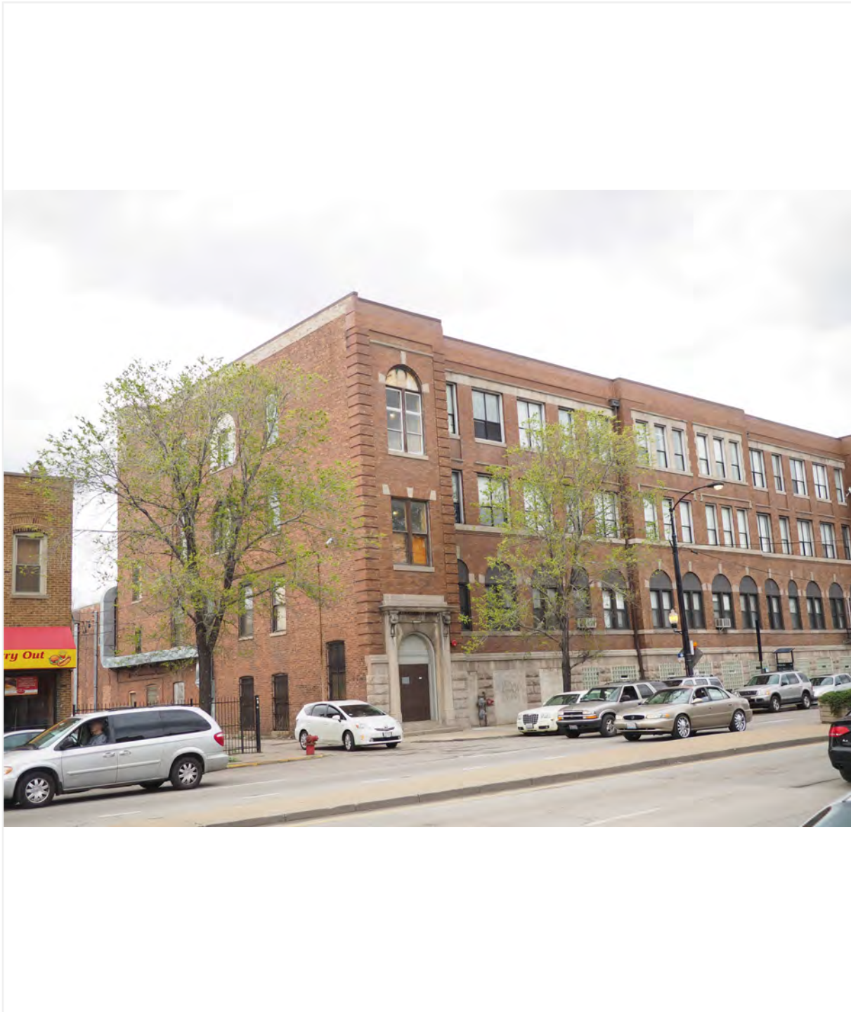
Facing northwest to south rear and east side elevations of main church and school building from South Western Avenue
