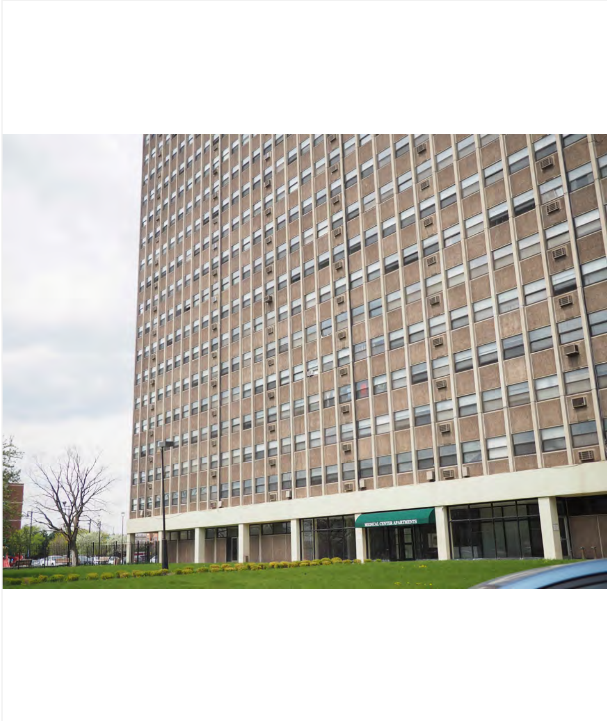
Facing northwest to south elevation entrance from West Ogden Avenue
