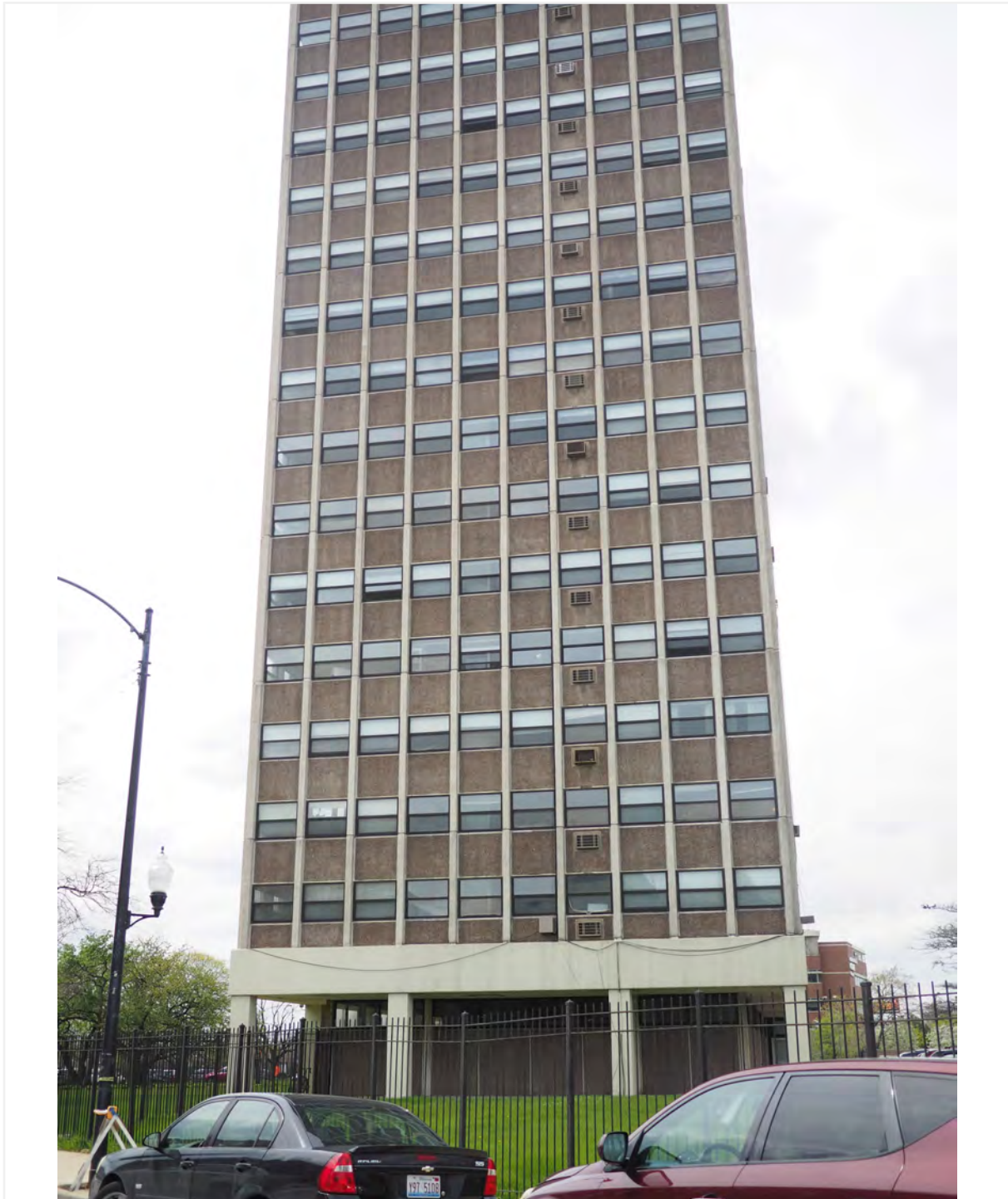
Facing west to east elevation from West Ogden Avenue
