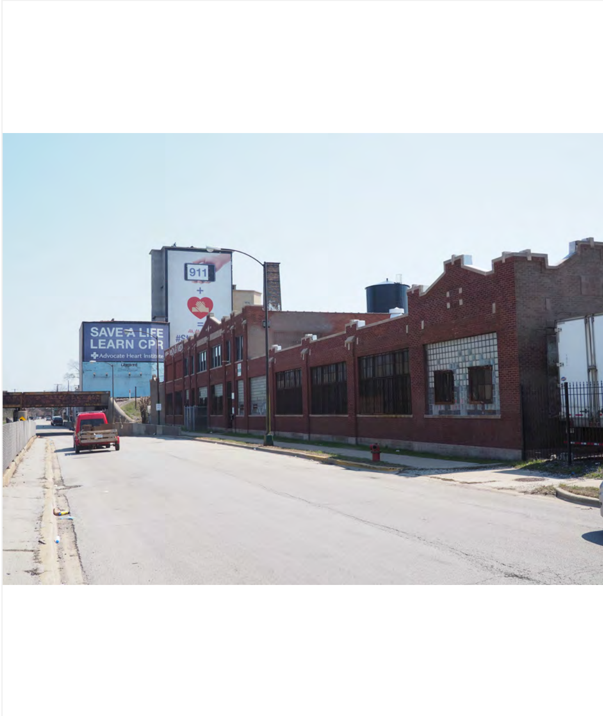
Facing southeast to north-facing facade and west side elevation from West Lexington Street
