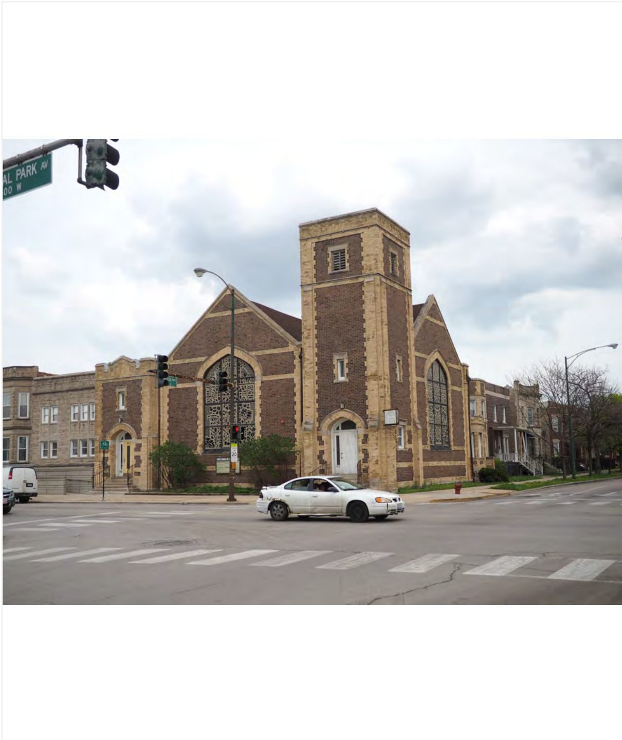
Facing northeast to south and west elevations from South Central Park Boulevard and West Congress Parkway
