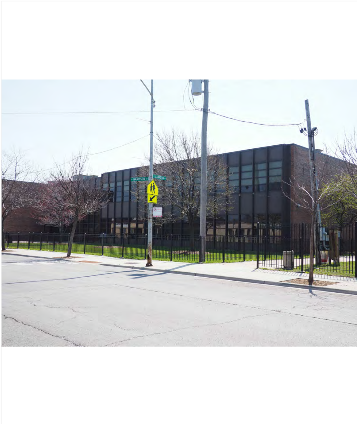
Facing southeast to north-facing facade and west side elevation from West Harrison Street
