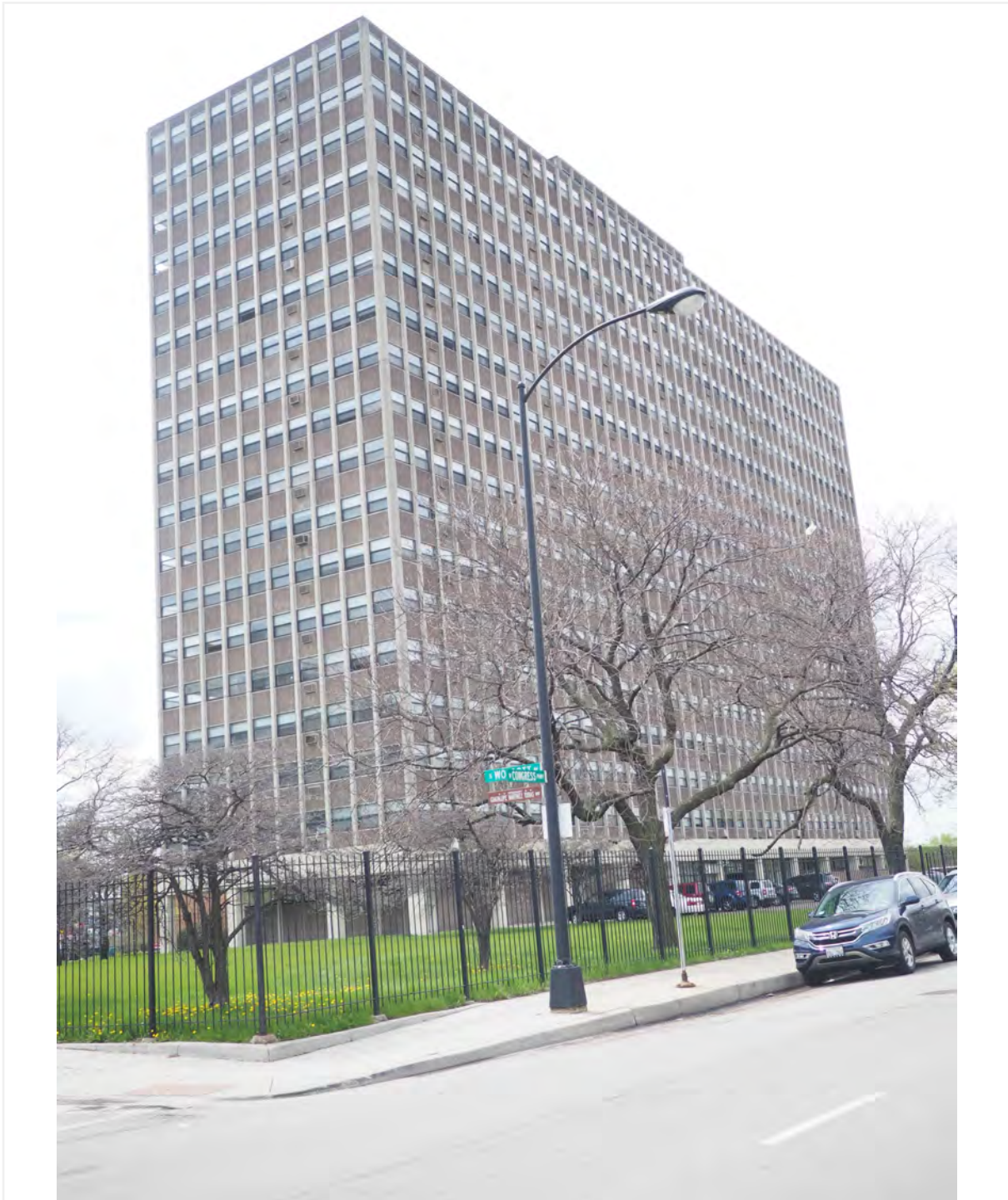
Facing southwest to north and east elevations from West Congress Parkway
