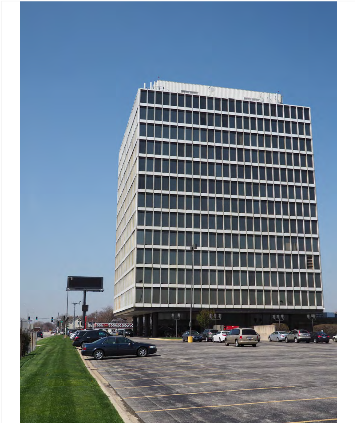
Facing northwest to south side and east rear elevations from West Harrison Street
