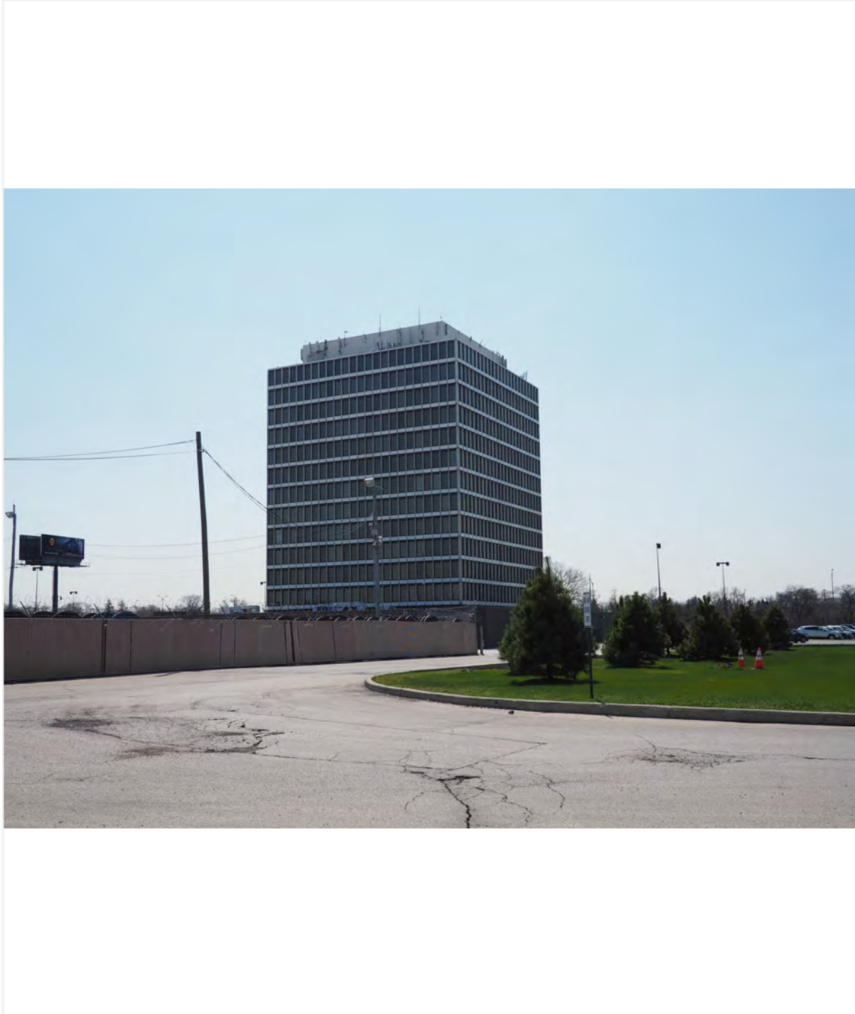
Facing southeast to north side and west-facing facade from South 1st Avenue
