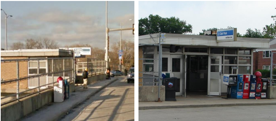
Figure 1-10. Narrow Sidewalks with Obstructions at Harlem and Oak Park Avenues
