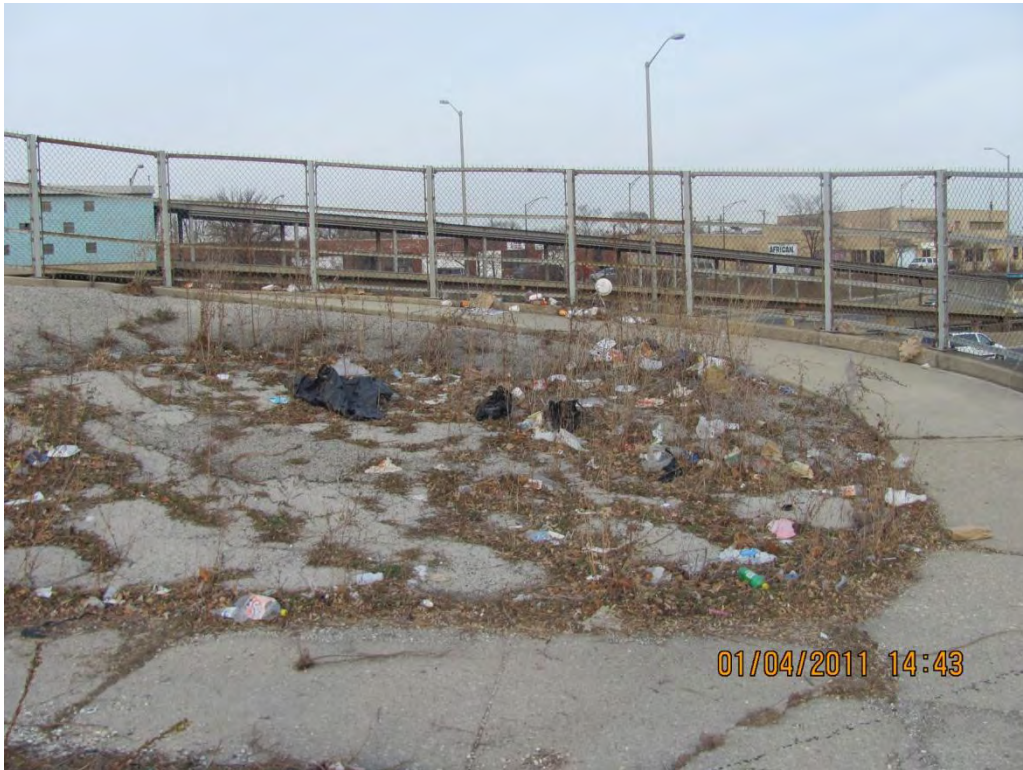
Figure 3-2 – Existing Lavergne Avenue pedestrian bridge over I-290
