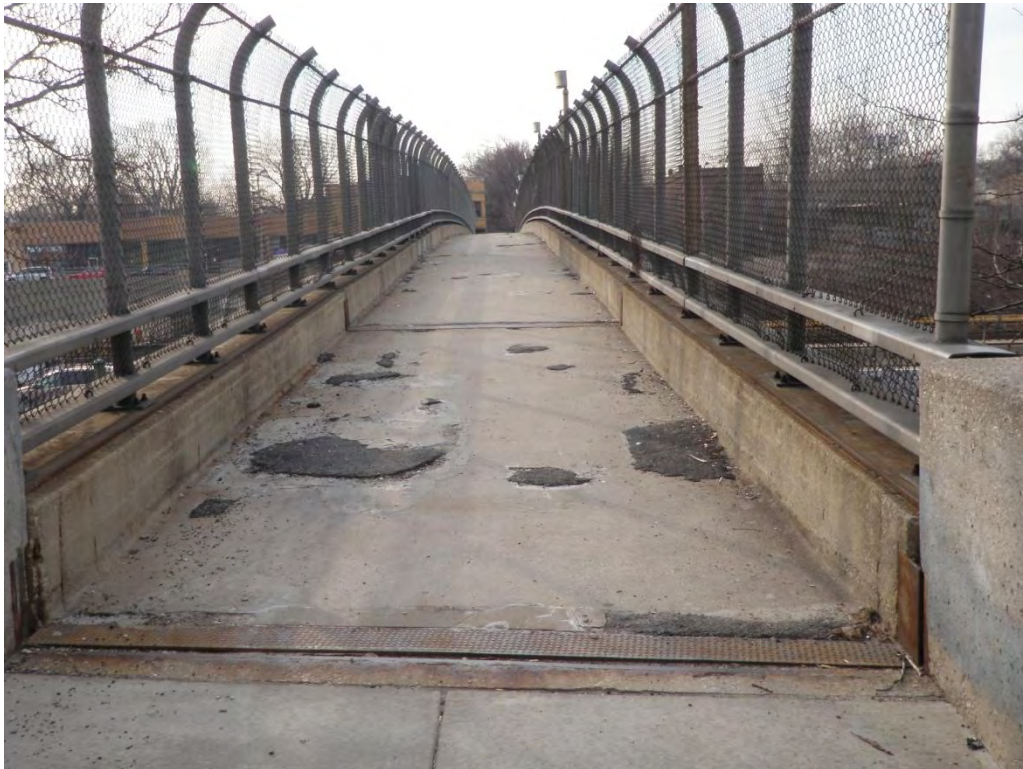
Figure 3-1 – Existing Home Avenue pedestrian bridge over I-290
