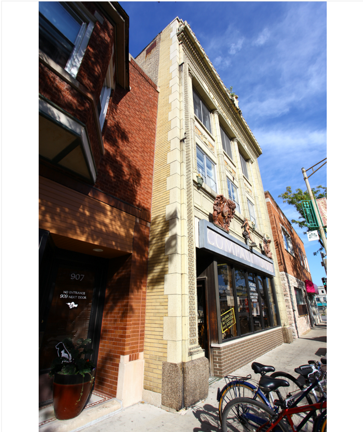
Facing northwest to east-facing facade and south side elevation from South Oak Park Avenue
