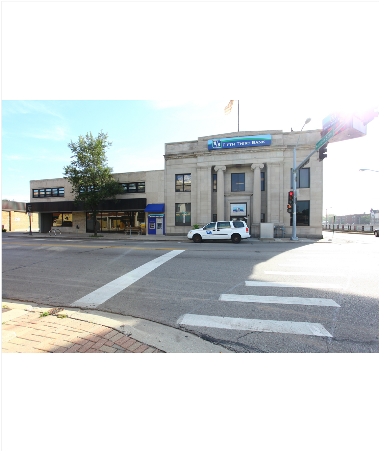
Facing east to west-facing facade of 1927 bank (right) and west-facing facade of ca. 1955 addition (left) from South Oak Park Avenue
