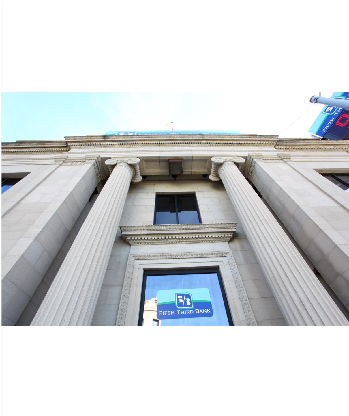
Facing east to west-facing facade portico from South Oak Park Avenue
