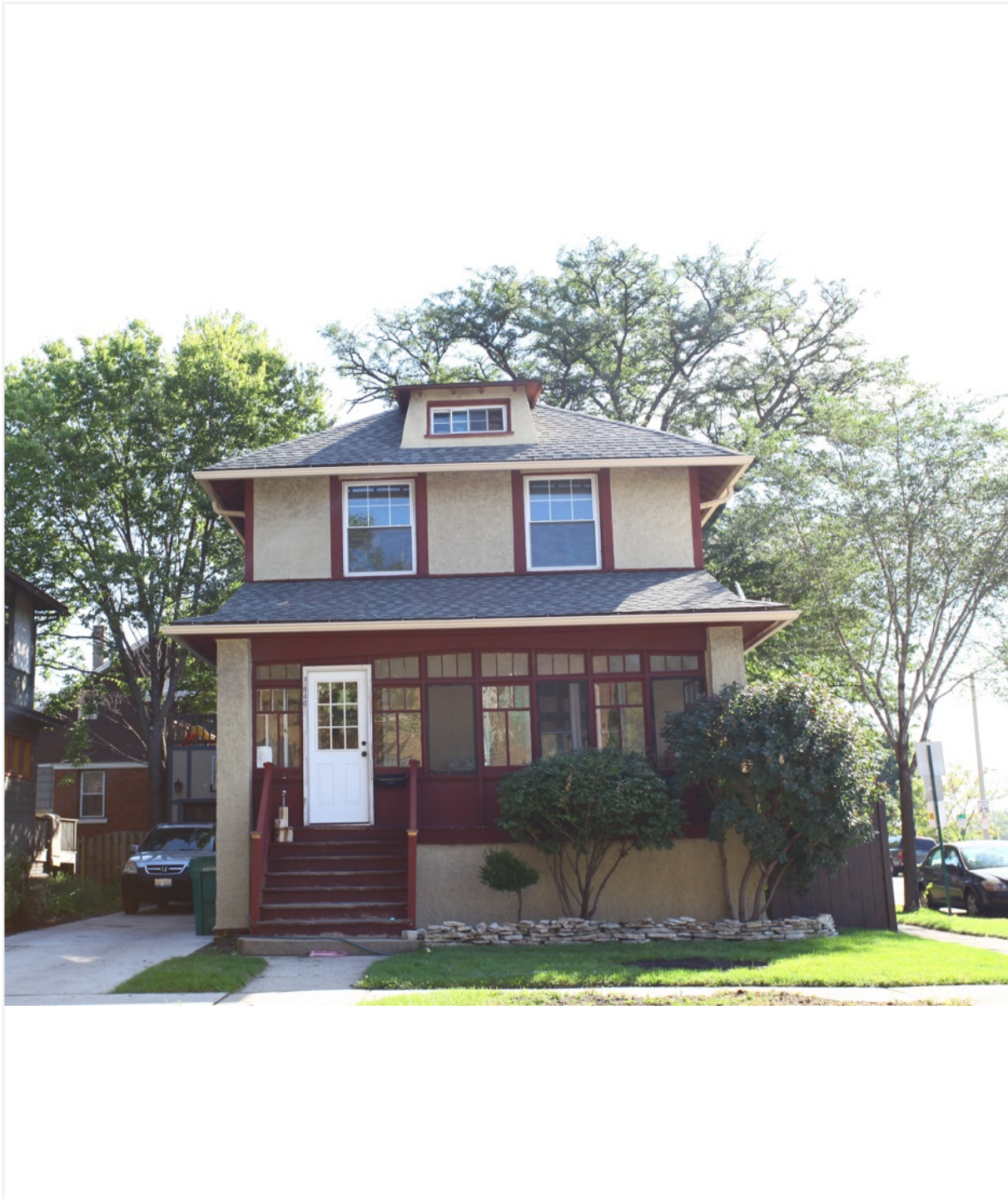
Facing east to west-facing facade from South East Avenue
