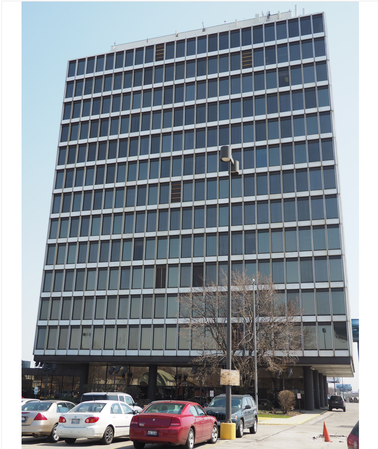
Facing east to west-facing facade from South 1st Avenue
