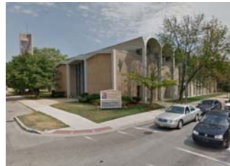
St. Eulalia Church 1851 S. 9 th Ave., Maywood Criterion C, Criteria Consideration A
