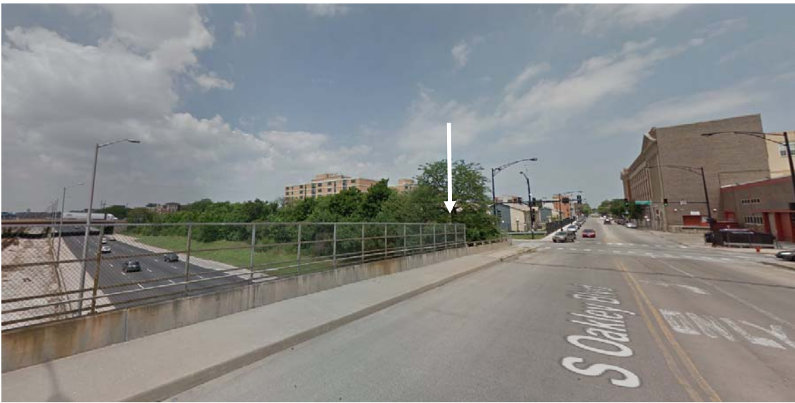
Figure 4-69. Crane Technical High School
