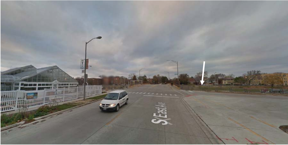
View north along South East Avenue toward Garfield Street and I-290 Preferred Alternative (at center), west side elevation (at left), and South East Avenue bridge (at center). B36 noise barrier location (arrow location, east of bridge) across I-290 along north interstate right-of-way, east of South East Avenue.
