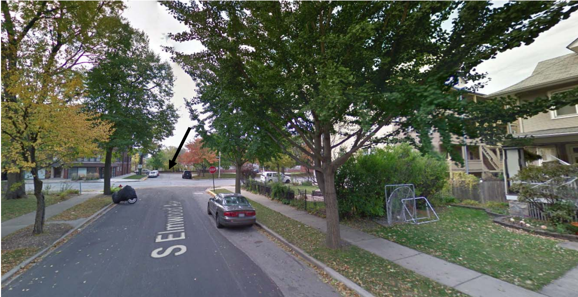
View southwest along South Elmhurst Avenue from within district boundaries and contributing buildings toward Harrison Street and I-290 Preferred Alternative (at center). B36 noise barrier location (arrow location, at center) along I-290 north right-of-way.
