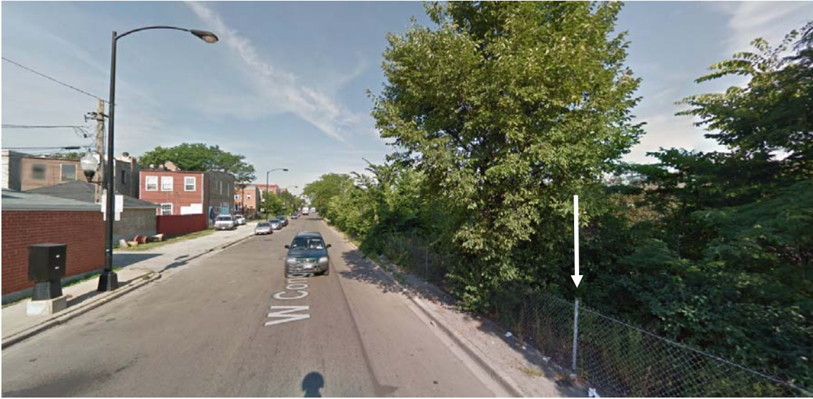
View west along West Congress Parkway from north district boundary at West Congress Parkway toward I-290 Preferred Alternative (at right) and contributing buildings along Claremont Avenue (at left, center). B75 noise barrier located along south I-290 right-of-way (arrow location at right) north of district.
