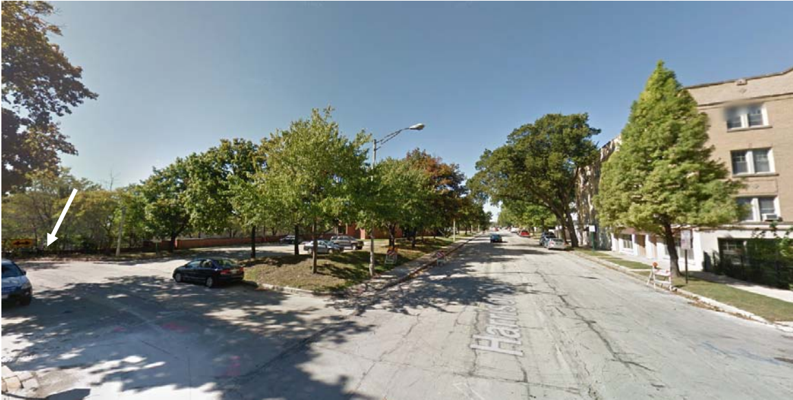
View southwest along Harrison Street at South Elmwood Avenue toward district's south NRHP boundary along Harrison Street, contributing building on west side of South Elmwood Avenue (at right), and I-290 Preferred Alternative (at left). B36 noise barrier location (arrow location, at left) along I-290 north right-of-way.
