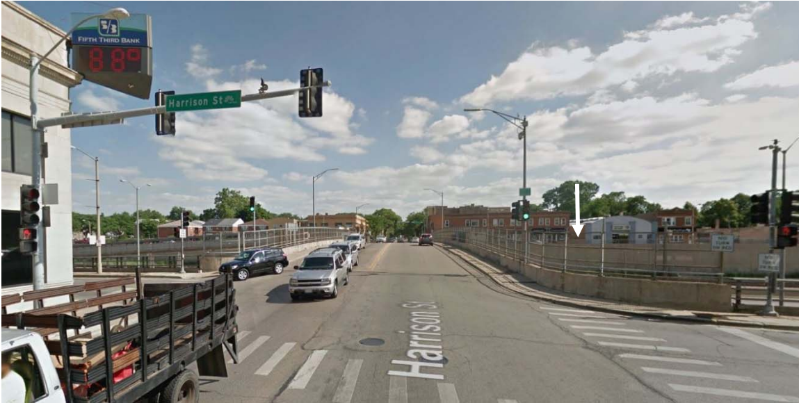
Figure 4-24. Suburban Trust and Savings Bank
