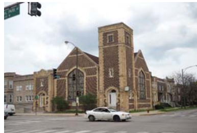
First Church of the Brethren 425 S. Central Park Blvd., Chicago Criterion C, Criteria Consideration A
