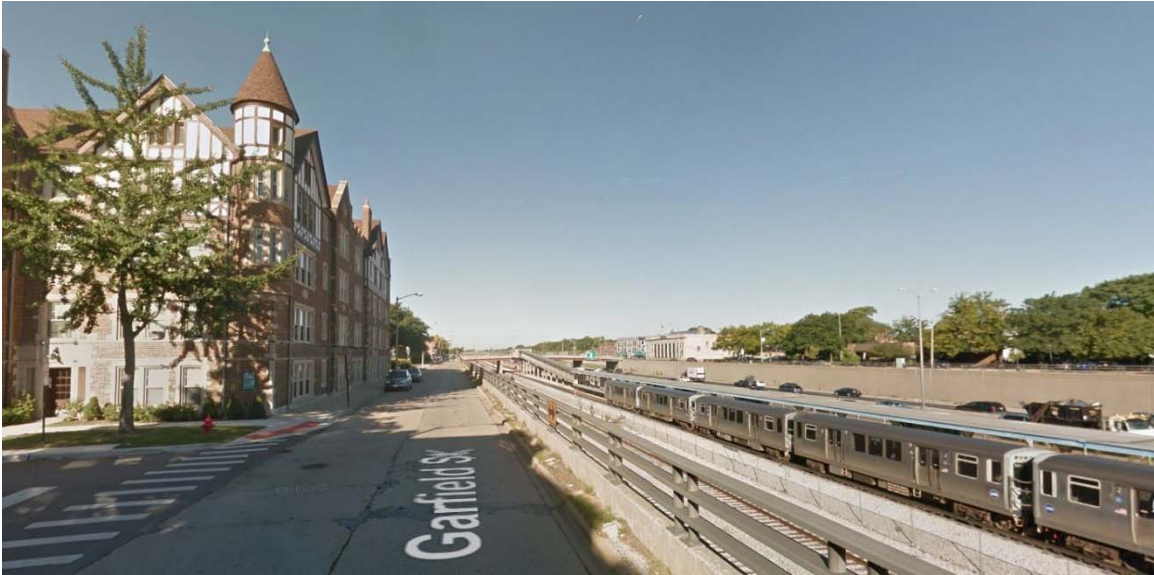
View west along Garfield Street at Welsey Avenue toward east-facing facade and north side elevation (at left) and I-290 Preferred Alternative (at right).
