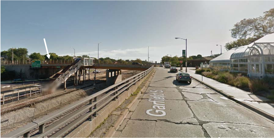
View east along Garfield Street toward north-facing facade (at right), South East Avenue (at center), CTA Blue Line station (at center, left), and I-290 Preferred Alternative (at left). B36 noise barrier location northeast (arrow location, at left behind bridge) across South East Avenue bridge and I-290 along north interstate right-of-way, east of South East Avenue.
