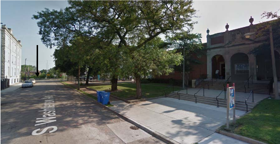
View northeast along South Washtenaw Avenue toward west-facing facade (at right) and I-290 Preferred Alternative (at center). B72 noise barrier location (arrow location, at left) along south I-290 right-of-way.
