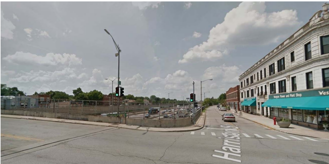
View west along Harrison Street across South Oak Park Avenue toward I-290 Preferred Alternative (at left) and building facade's south elevation and southeast corner (at right). B33 noise barrier location at far left, along existing I-290 south right-of-way.
