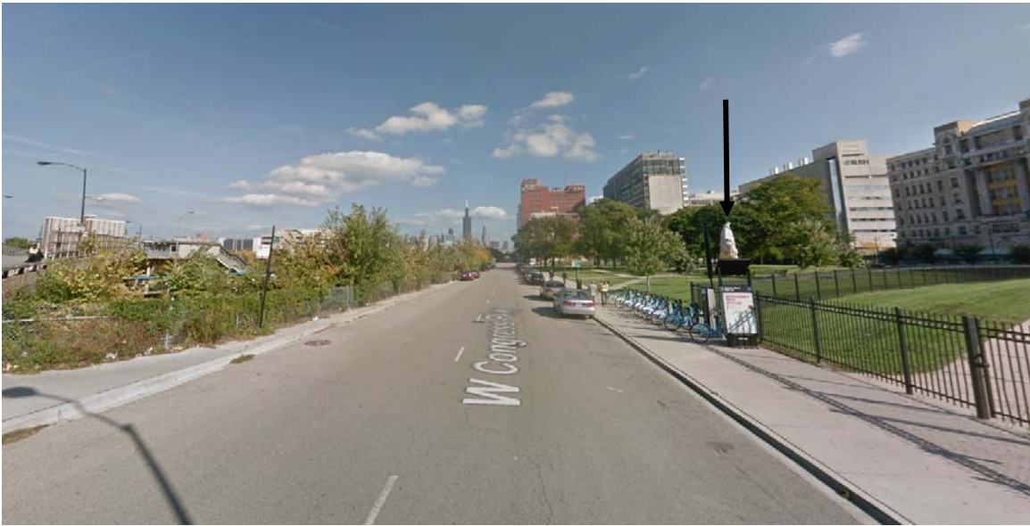
View east along West Congress Parkway from West Ogden Avenue toward I-290 Preferred Alternative (at left), Louis Pasteur Memorial (arrow location at center, right), and Cook County Hospital Administration Building (at right). B83 noise barrier location along south I-290 right-of-way and existing fence (at left).
