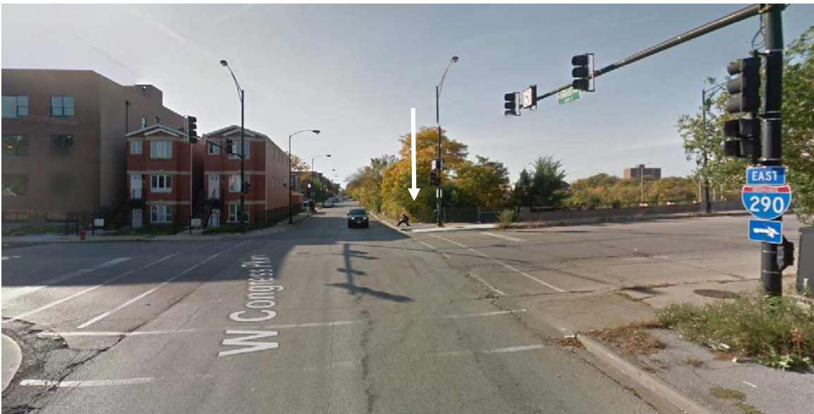
View west along West Congress Parkway from at South Oakley Boulevard toward district's northeast NRHP boundary at South Oakley Boulevard and West Congress Parkway (at left) and I-290 Preferred Alternative (at right). B75 noise barrier located along south I-290 right-of-way (arrow location at right center) north of district.
