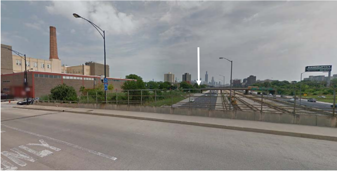
Figure 4-68. Crane Technical High School
