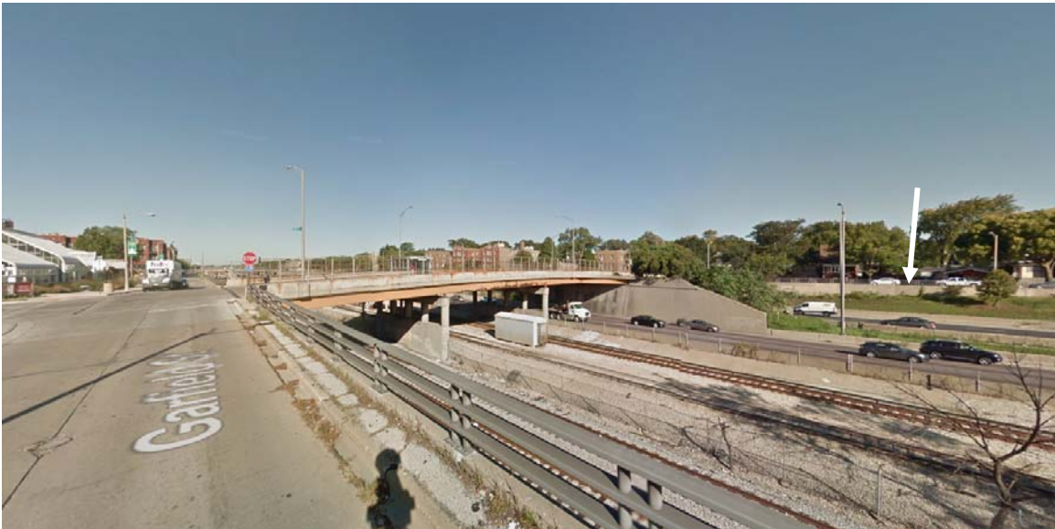
View northwest along Garfield Street toward Oak Park Conservatory (at left), I-290 Preferred Alternative (at center), and South East Avenue bridge (at center). B36 noise barrier location (arrow location, at right) along I-290 north right-of-way, east of South East Avenue.
