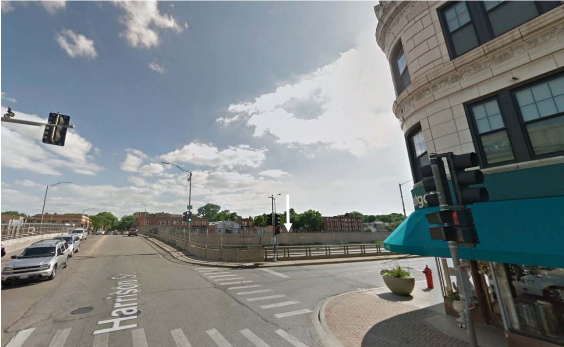
View south along South Oak Park Avenue at Harrison Street intersection toward South Oak Park Avenue bridge (at left), I-290 Preferred Alternative (at center) and building facade's east elevation and southeast corner (at right). B33 noise barrier location at center (arrow location), along existing I-290 south right-of-way.
