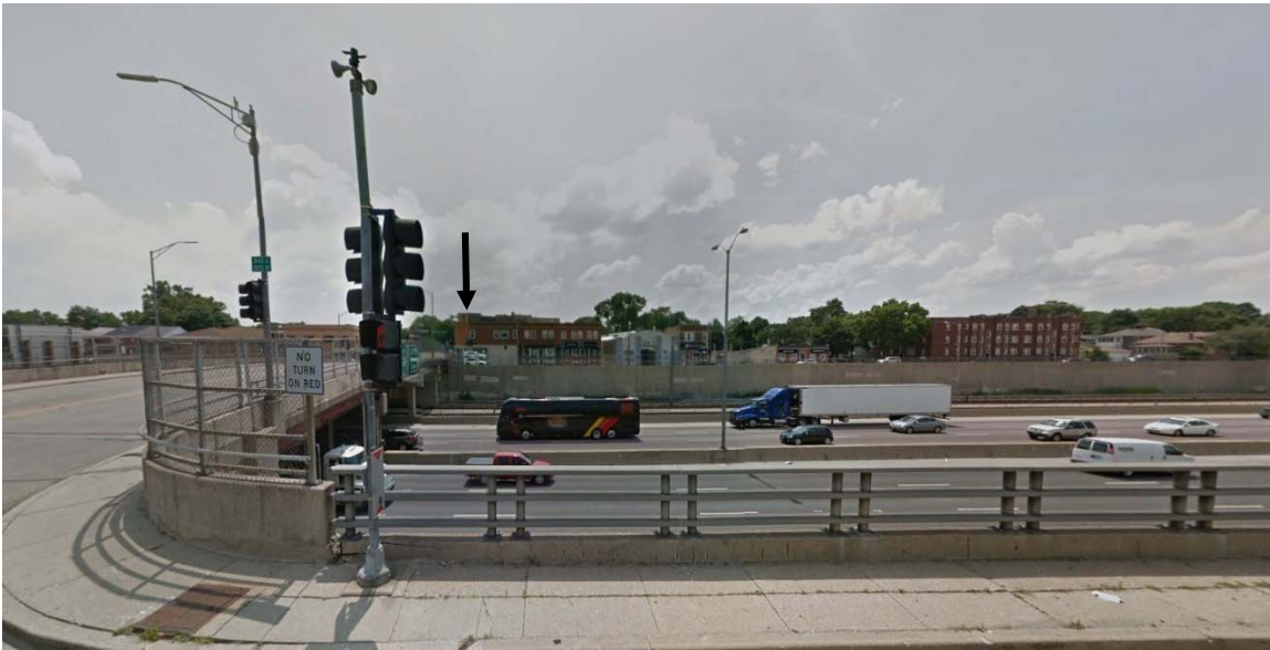
View southwest from Harrison Street toward T.A. Holm Building (arrow location, behind red brick building) and I-290 Preferred Alternative. B33 noise barrier location at center, along south I-290 right-of-way.
