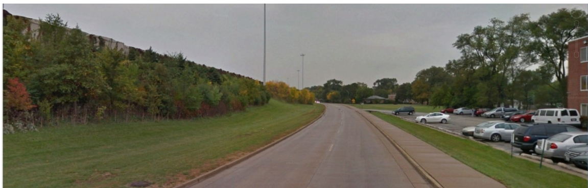
View looking southwest of planted embankment and noise barrier along north frontage road proximate to Hillside Drive. Planting is between noise barrier and frontage road.
