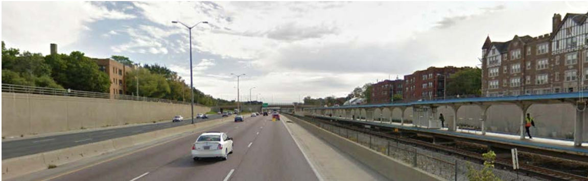
Retaining walls (left), CTA facilities, and mid-rise adjacent housing structures (right) contain viewshed of the Project Corridor east of South Oak Park Avenue along the eastbound mainline.
