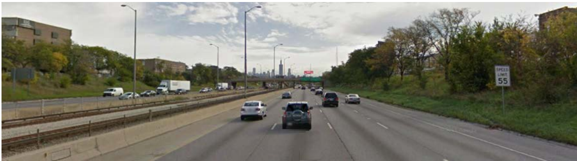
Figure 3-81. I-290 Mainline View East of South Central Park Boulevard
