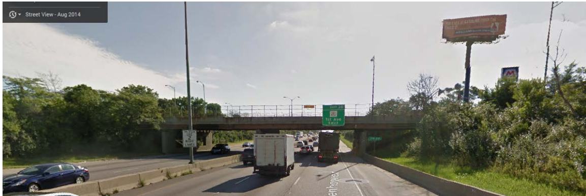
Figure 3-72. Roadway View at 17 th Avenue
