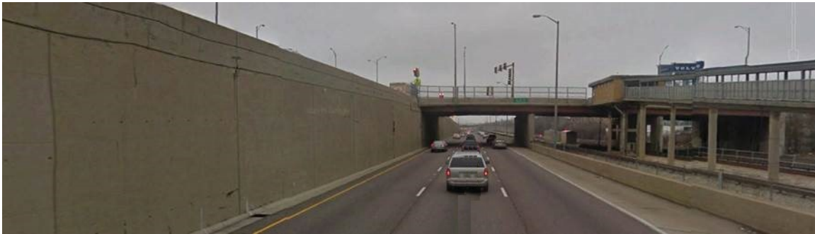
Center on/off-ramp walls (left) and CTA facilities (right) frame view along eastbound I-290 at Harlem Avenue.
