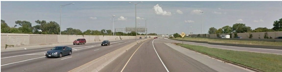
Existing noise barriers screen views to adjacent residential neighborhoods in the western portion of the Study Area.
