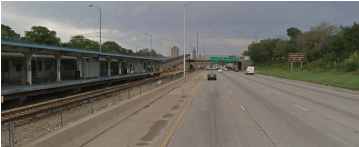
Figure 3-82. I-290 Eastbound West of South Pulaski Road
