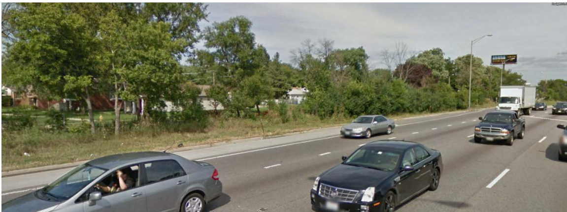
Variability in the density of right-of-way planting allows occasional views to adjacent residential neighborhoods. View looking north to residences north of freeway proximate to South 21 st Avenue.
