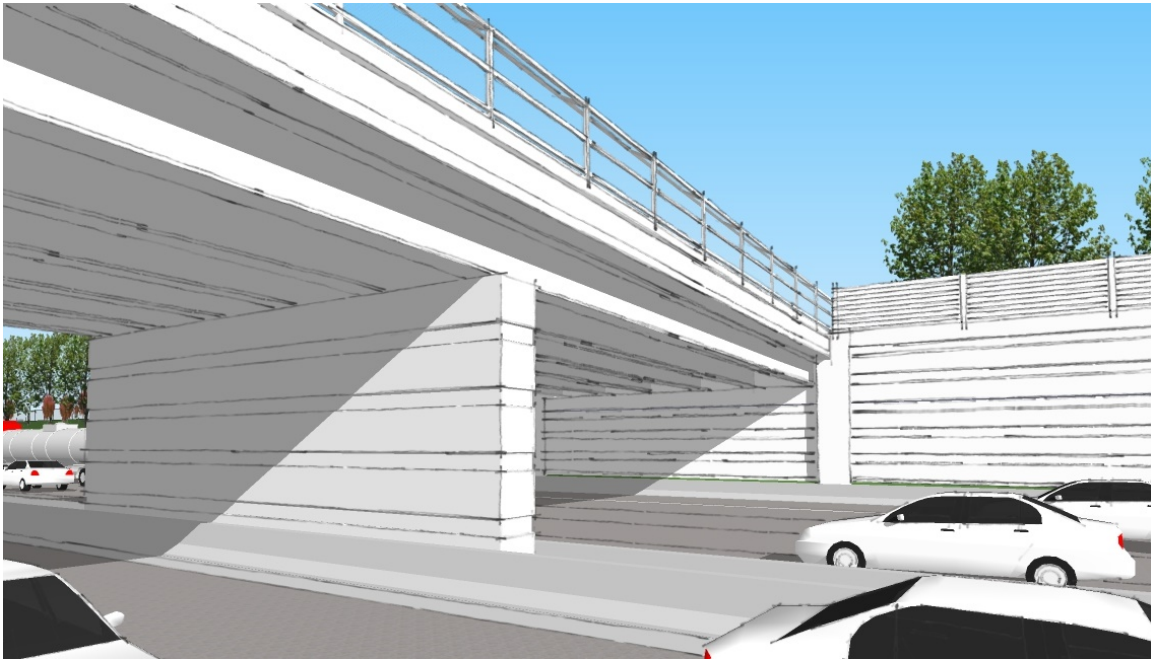
Image of cross-street overpass (left), retaining wall, fencing, and landscape (right) along north I-290 right-of-way at Ridgeland Avenue. Note: Landscape is at frontage road height and readily visible from the adjacent neighborhood beyond.
