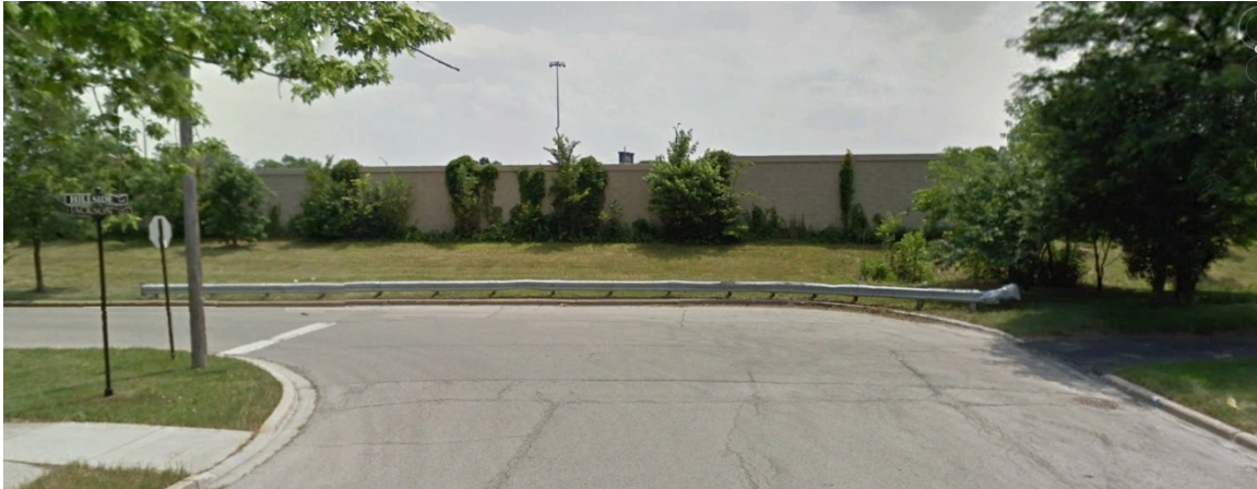
View of freeway right-of-way and associated noise barrier at Hillside Avenue/Jackson Boulevard north of freeway.
