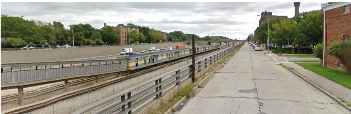
View of the Project Corridor looking north through vehicle barrier adjacent to Garfield Street.
