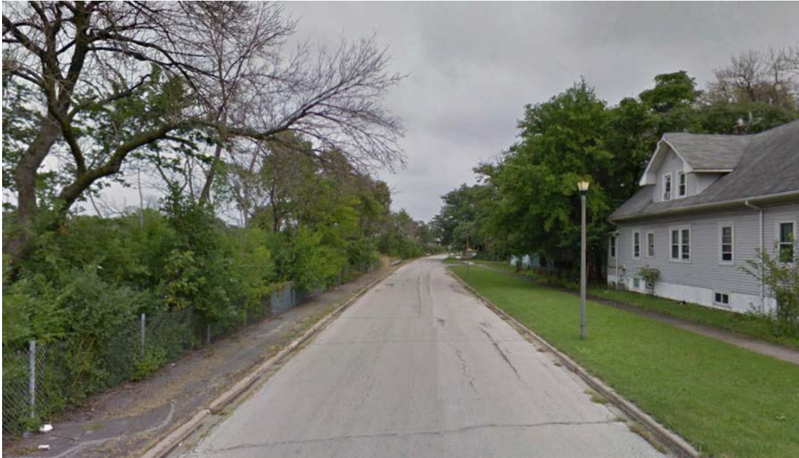
Figure 3-91. View of Bataan Drive near 23 rd Avenue
