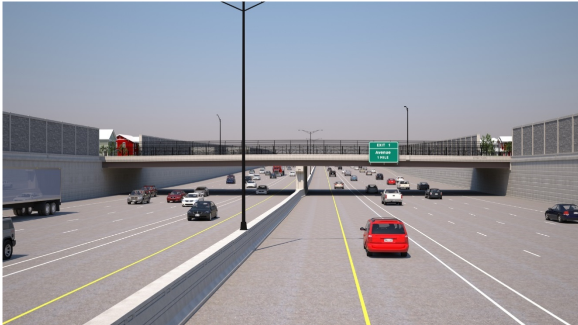
Reconstructed freeway with perimeter retaining walls, noise barriers, and overpass with decorative barrier and metal fencing.
