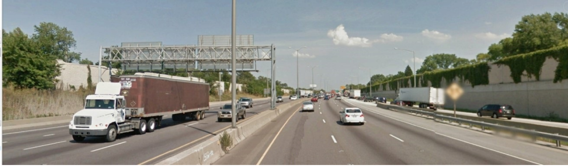
Figure 3-68. Mainline Roadway View – Retaining and Noise Barriers
