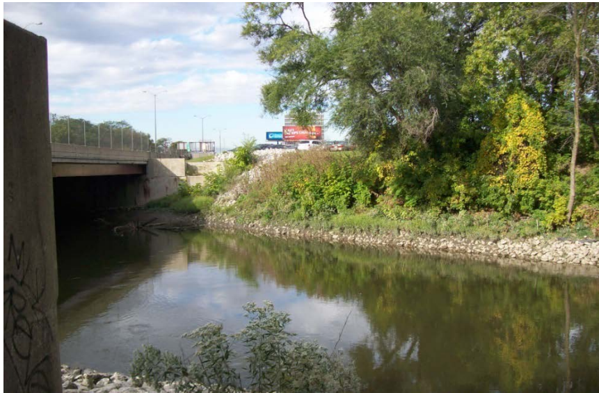
Figure 3-56. Des Plaines River, north of I-290
