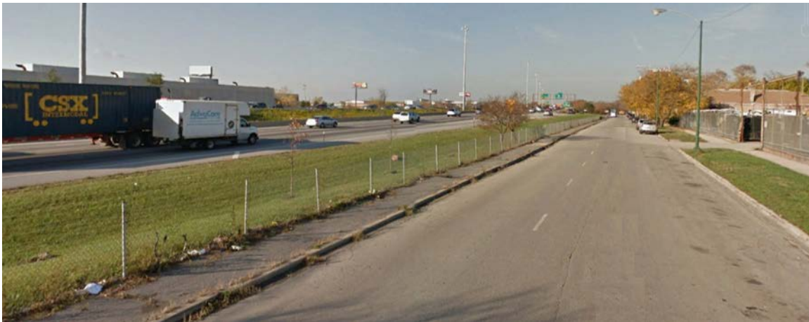
Right-of-way with turf planting only along westbound mainline at West Flourney Street, west of South Lockwood Avenue.
