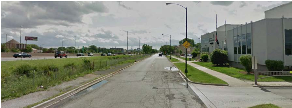
Figure 3-101. View along West Lexington Street
