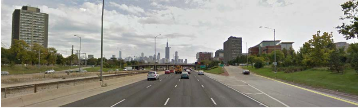
Figure 3-80. I-290 Eastbound near South Damen Avenue
