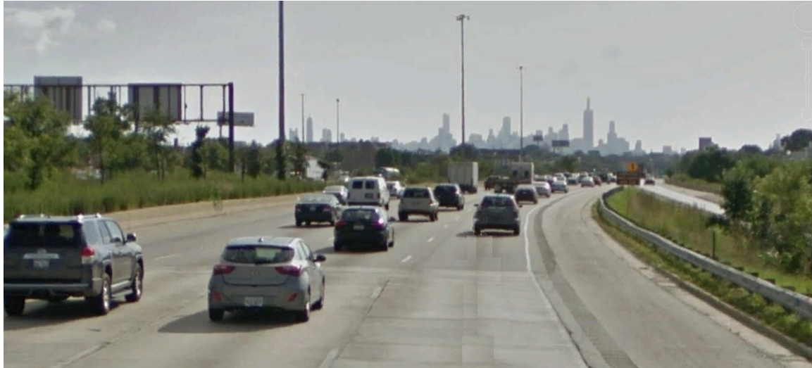
Figure 3-78. I-290 Eastbound East of South Central Avenue
