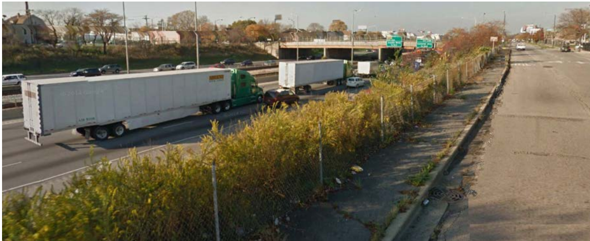
Fencing and hedge row planting along right-of-way West Flourney Street, East of South Laramie Avenue.
