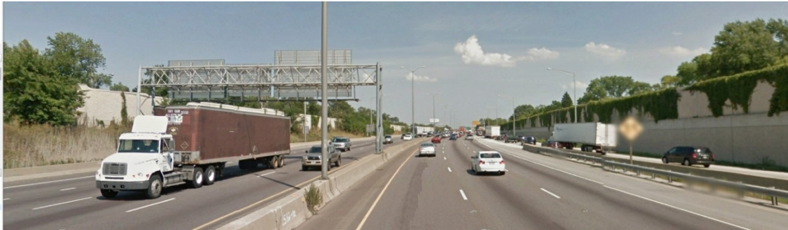
Figure 3-68. Mainline Roadway View – Retaining and Noise Barriers
