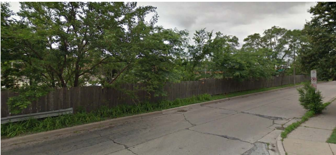
Vegetation in I-290 right-of-way behind wood screen fence along Harrison Street frontage road near Kenilworth Avenue.
