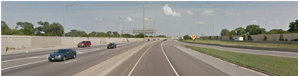
Existing noise barriers screen views to adjacent residential neighborhoods in the western portion of the Study Area.
