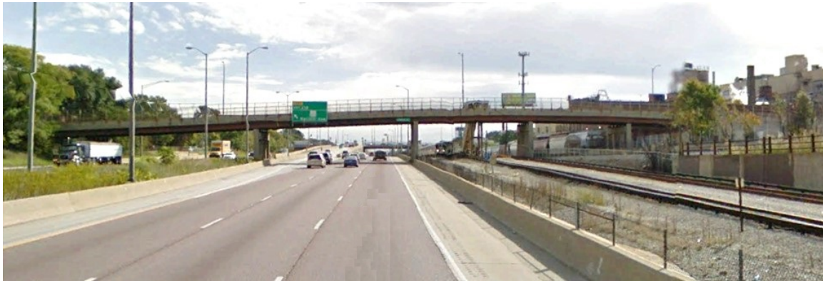
A common visual element, CTA facilities and CSX rail track, are visible south of the Project Corridor proximate to Circle Avenue.
