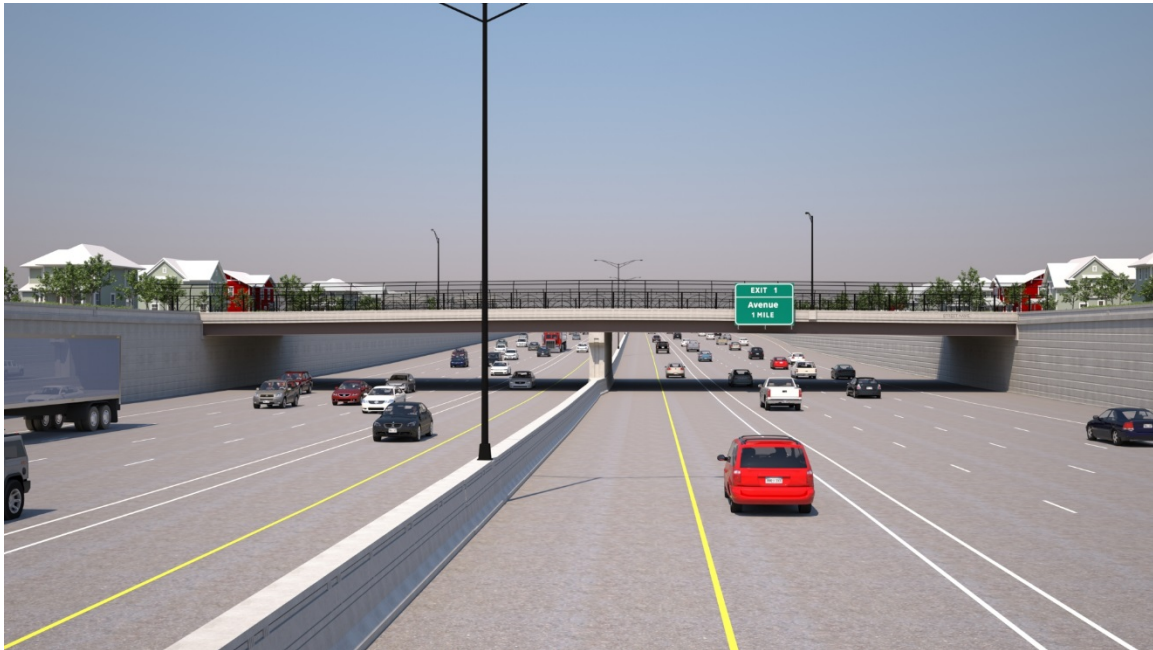
Reconstructed freeway with perimeter retaining walls and decorative fencing on overpass.
