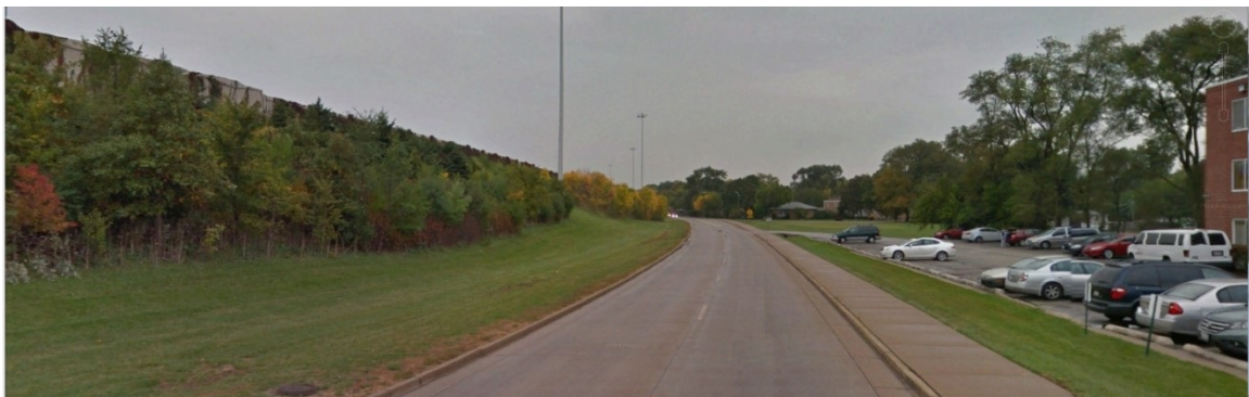
View looking southwest of planted embankment and noise barrier along north frontage road proximate to Hillside Drive. Planting is between noise barrier and frontage road.
