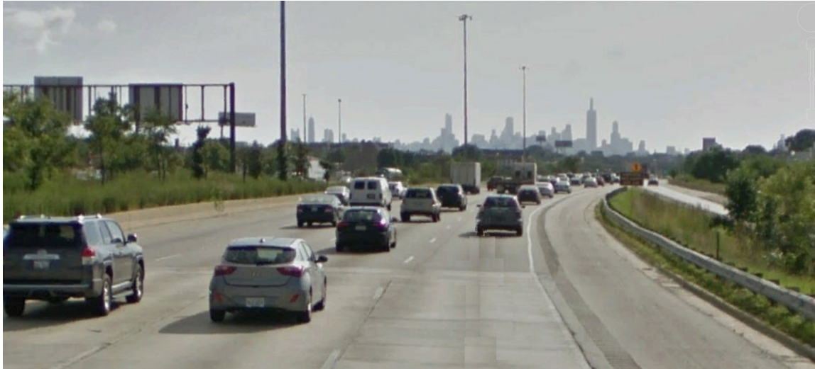
Figure 3-78. I-290 Eastbound east of South Central Avenue
