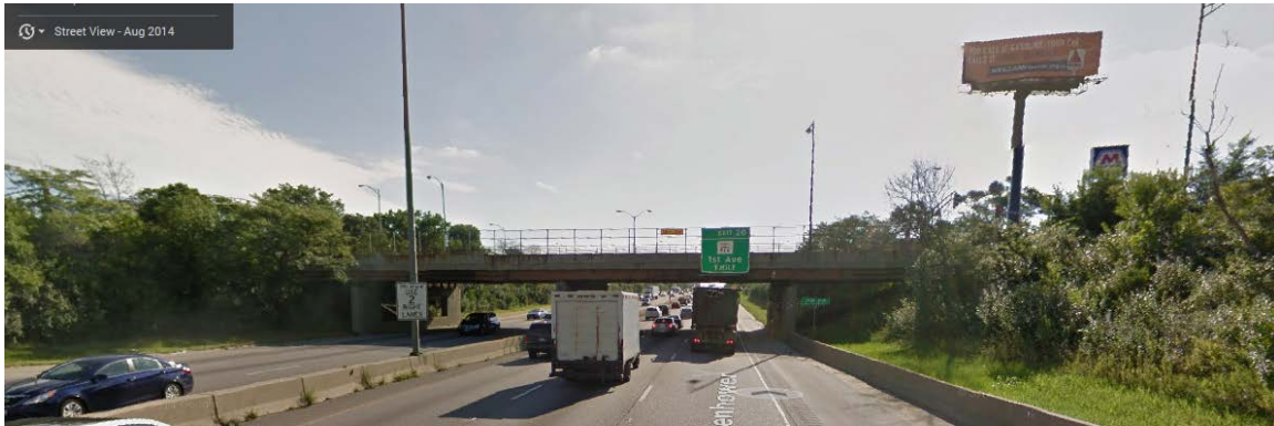
Figure 3-72. Roadway View at 17 th Avenue
