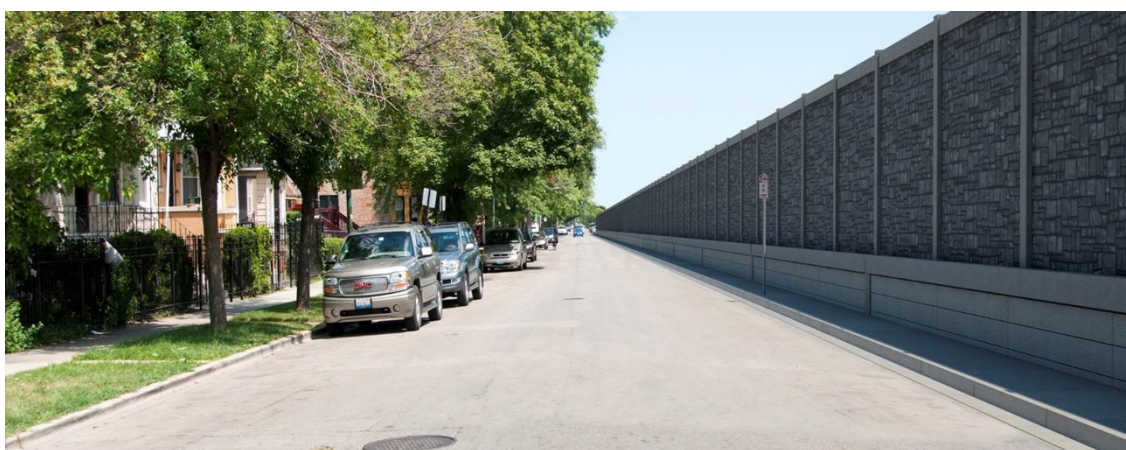
Simulation of potential noise barrier as viewed from Congress Street and Keeler Avenue, City of Chicago.
