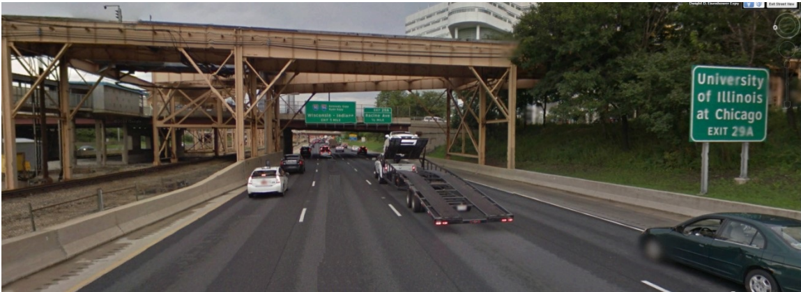
Figure 3-83. Eastbound Mainline View West of South Paulina Street
